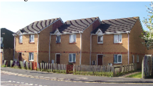
Lower Well Road (subject to flooding)
