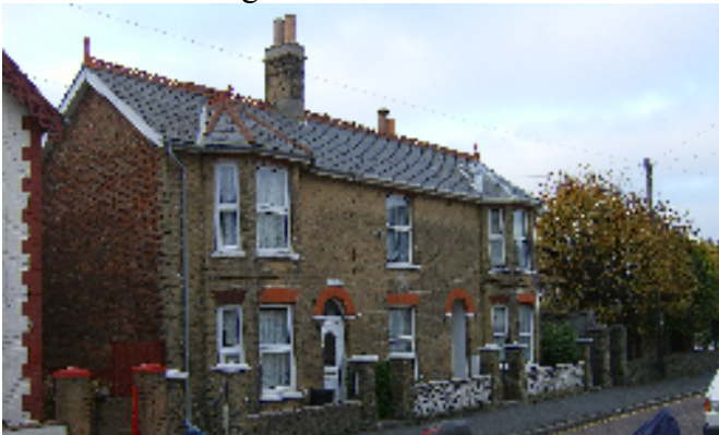
Osborne Road – ridge tiles /finials
