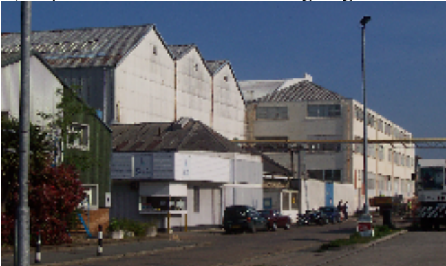
Columbine buildings, Castle Street
