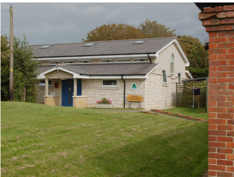
Brighstone Scout, Guide and Community Centre (KS)
