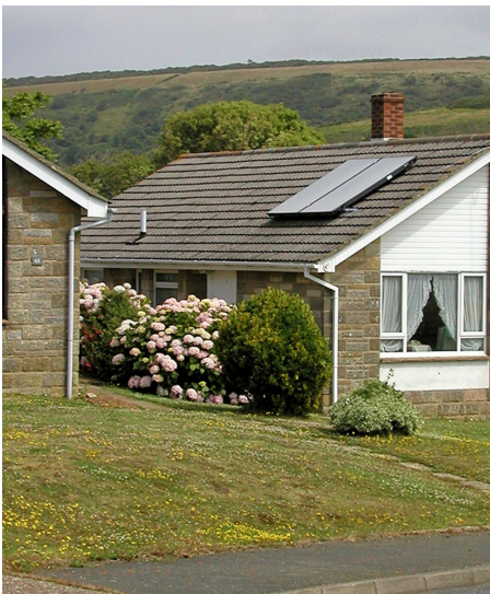
Solar Water Heating (DWM)
