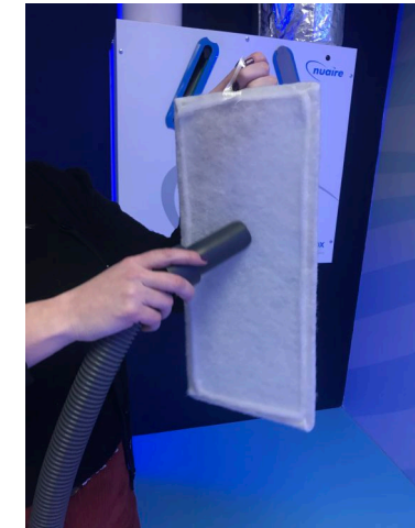
MVHR filters are easy to remove and clean, clean filters improve energy efficiency
