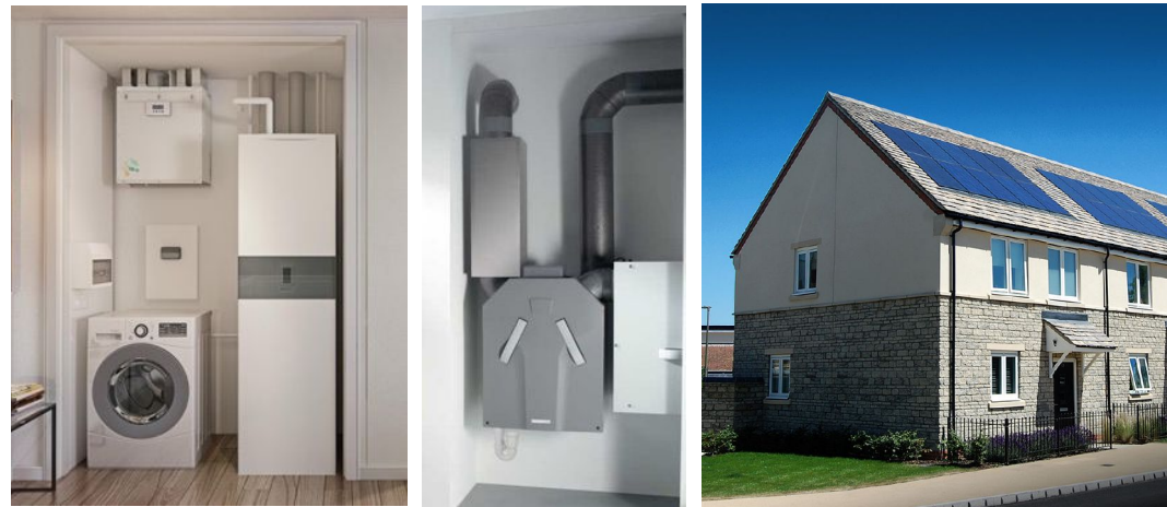
Technology that drives down energy consumption is easily available. Designers and contractors must however allow for these systems early-on in scheme conception and pay close attention to their installation, commissioning and maintenance. Allowing space on floor plans from an early point in design is crucial. The above images show the integration of (from left to right) an individual heat pump, a mechanical ventilation system with heat recovery, and roof mounted photovoltaics.
