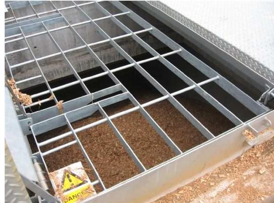
Delivering into an underground store with 30m<sup>3</sup> hook lift bin (South East Wood Fuels)
