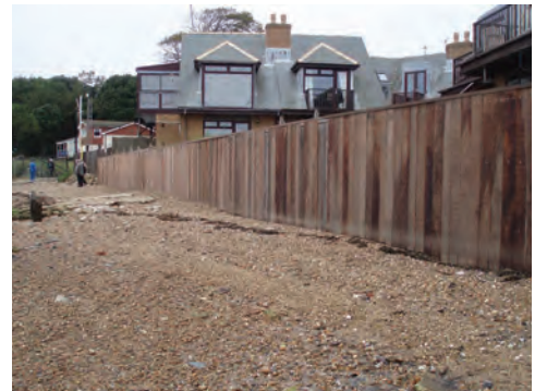
Timber Clad Sheet Pile Wall
