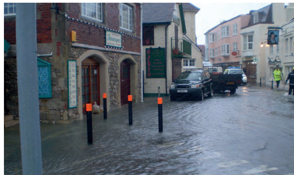
Tidal flooding in Quay Street Yarmouth (March 2008)
