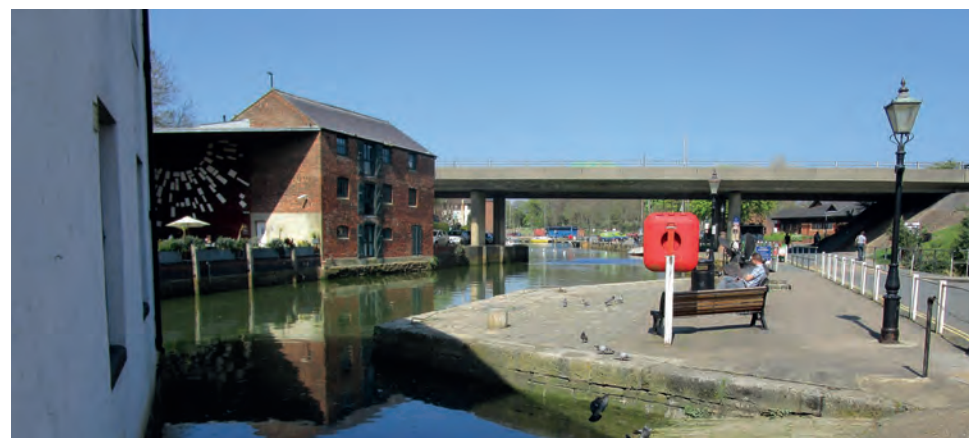
Quay walls of Newport Harbour
