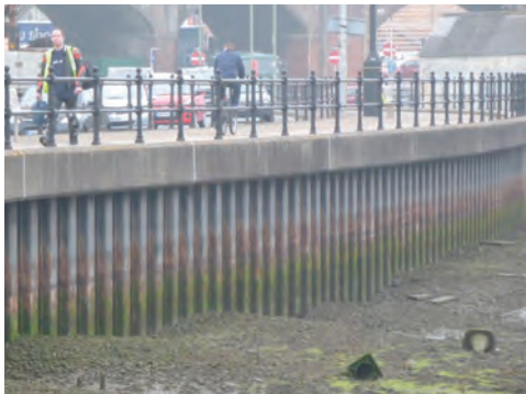
Steel Sheet Piling
