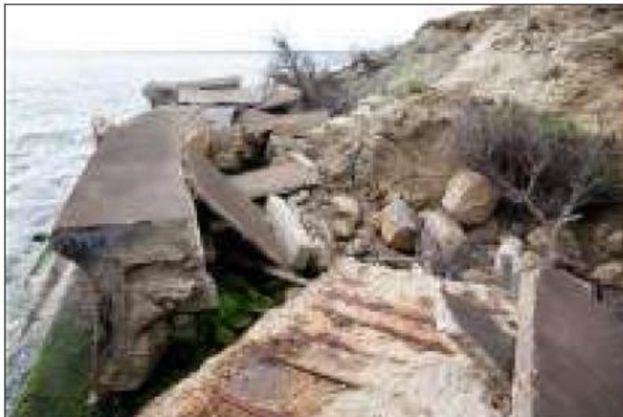
The storm hit sea wall at West Wight. Picture by Paul Blackley.
