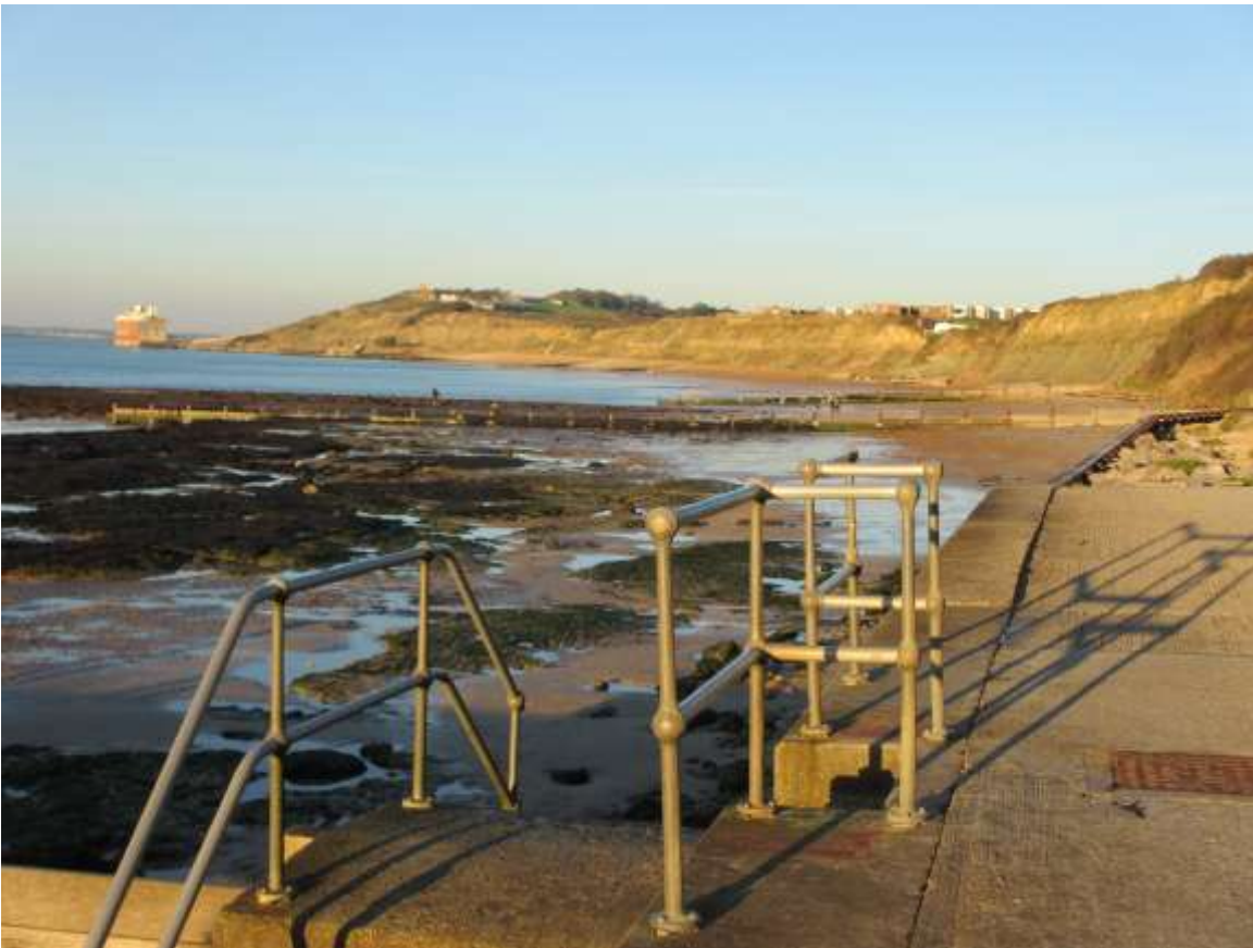
Colwell Bay, showing the transition from the defended to undefended coast and showing exposed rock ledges in the foreshore, looking north across groynes towards Fort Albert, in 2012.
