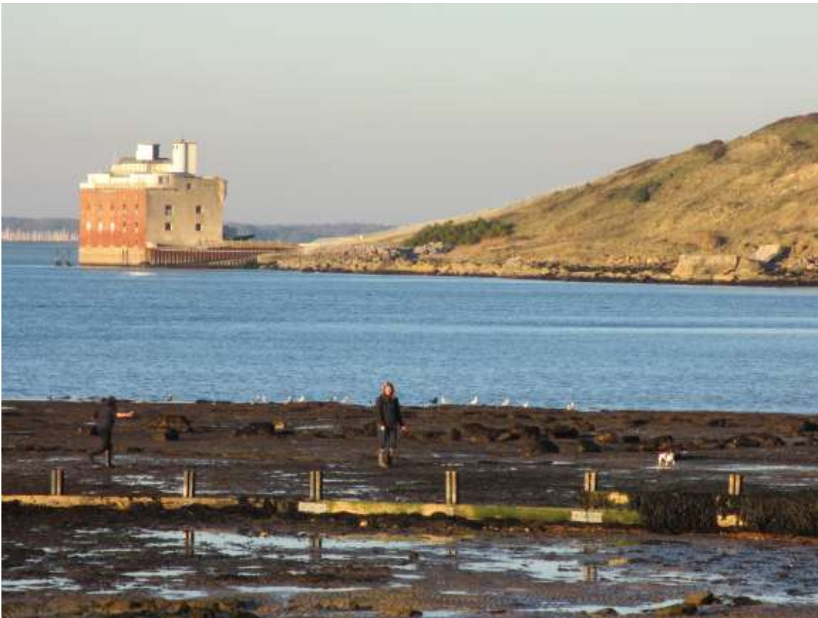
Fort Albert, at the northern end of Colwell Bay, 2012
