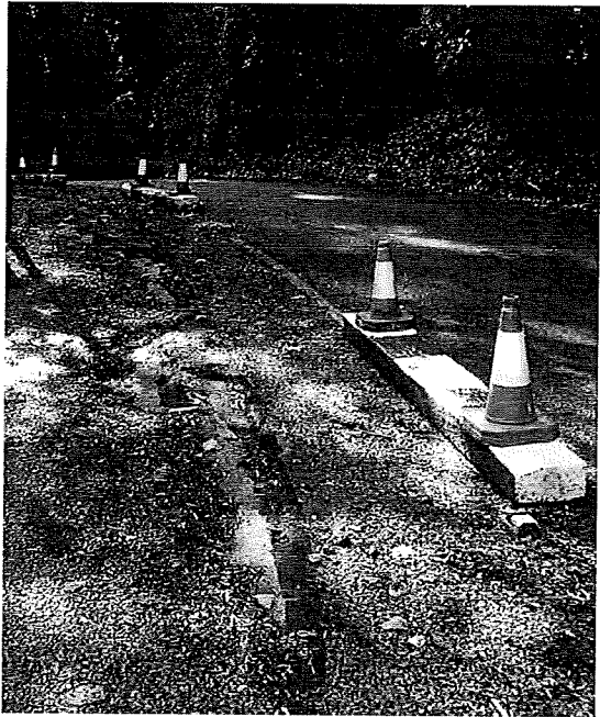
Plate 3: Crack damage observed in the westbound carriageway, Area 3 Undercliff Glen
