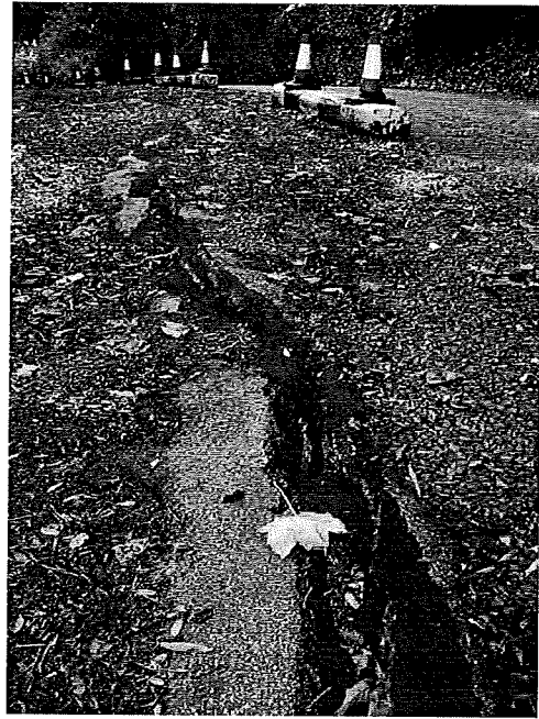
Plate 3: Crack damage observed in the westbound carriageway, Area 3 Undercliff Glen
