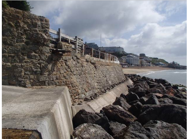
Spyglass - Stone masonry wall
