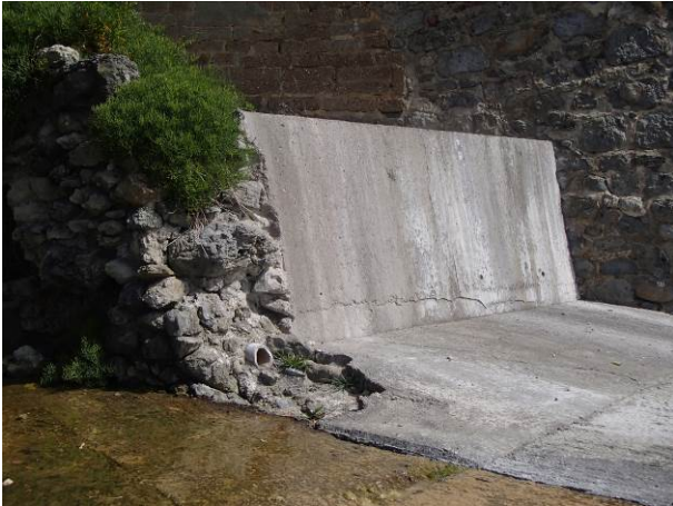
Old outfall pipe – no running water
