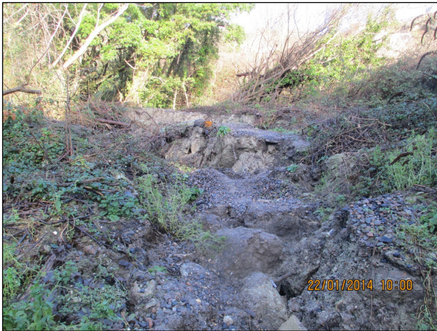
Figure 1c. Site 10 Caravan Park Geological Failure: Large tension cracks approximately 100m downslope of the site.
