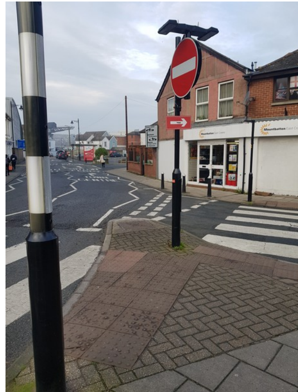
Figure 33: A pinch point at the entrance to Ferry Road in the one-way system leaves little space for a shared use cycle path
