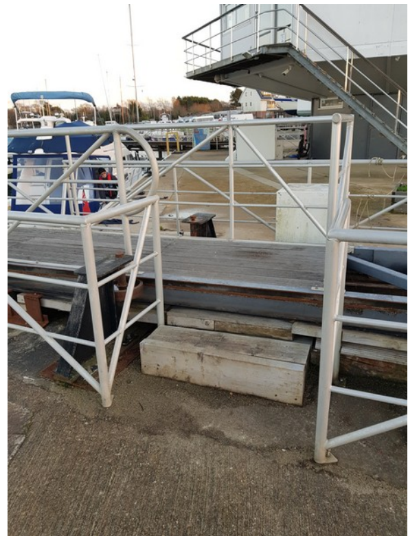
Figure 23: Steps to the lock gate access at Island Harbour
