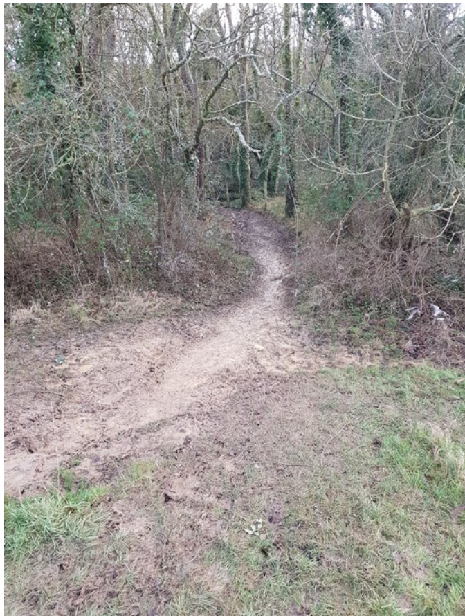
Figure 4: Part of public footpath CS24 from St Mildred's Church to Folly Inn, part of route IOW 10. Photo taken in January 2022, when mud on the slope into the woods made the path treacherous
