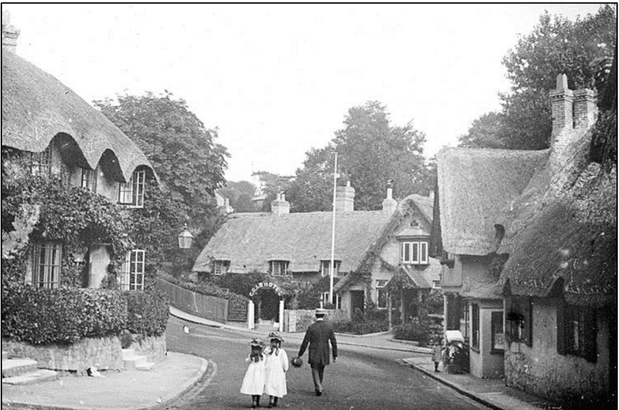
Shanklin Old Village. A view of Shanklin old village, the Crab Hotel can be seen in the background. 1898
