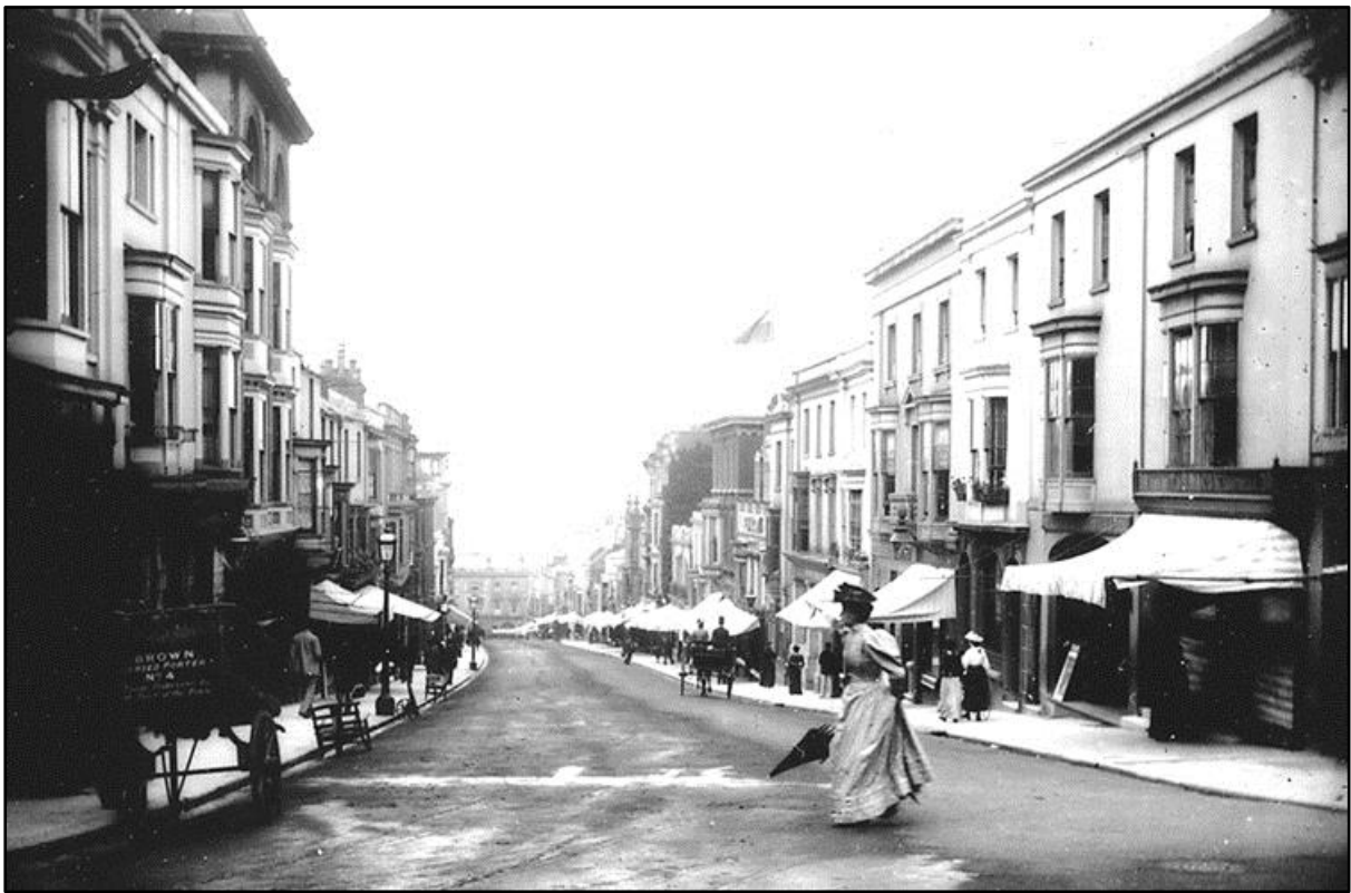
Ryde - Union Street. A view of Union Street, Ryde. On the extreme left is the cart of porter C. Brown, licenced no.4, luggage conveyed to any part of town. Circa. 1900-1910
