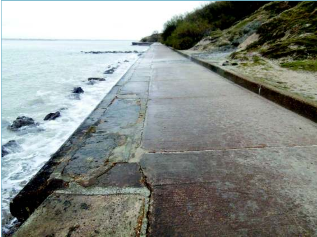
Figure 8.2: Defence Section 1 South – No current signs of seawall movement
