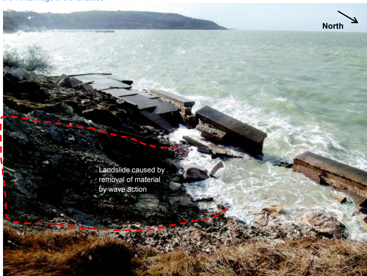
Figure 4.4: Landslides of the frontal ridge due to removal of toe support by the waves. Photo taken looking SW from the frontal ridge of the landslide.
