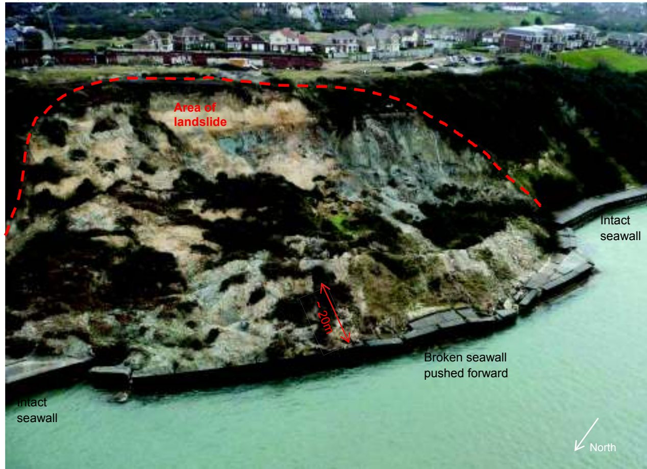
Figure 2.3: Photograph of the landslide and the distance moved by the seawall.
