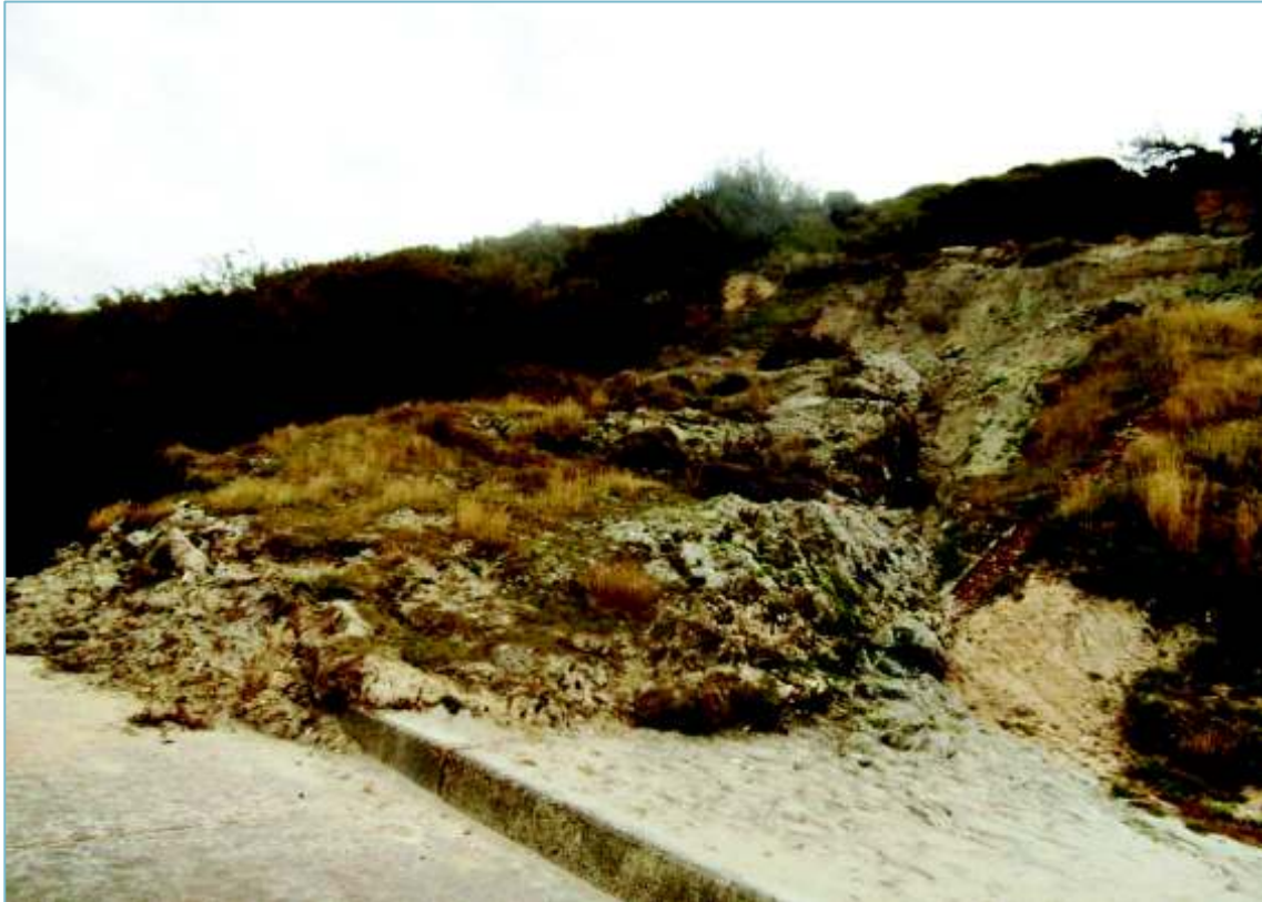
Figure 8.4: Defence Section 1 - Minor landslips at Totland Bay, spilling on to Promenade.
