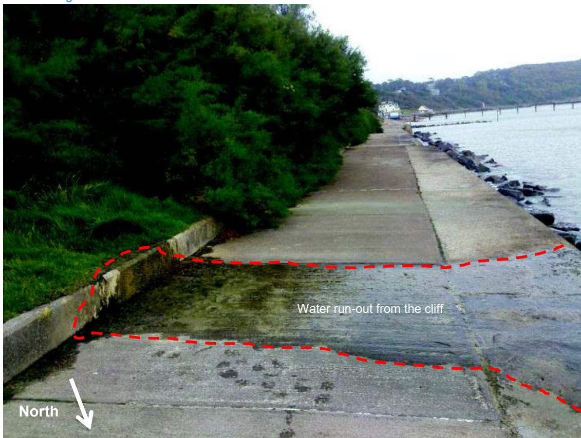
Figure 5.2: The run out of water in the section south of the landslide observed on 22 nd October 2013. This photo is taken looking south towards Totland Pier.
