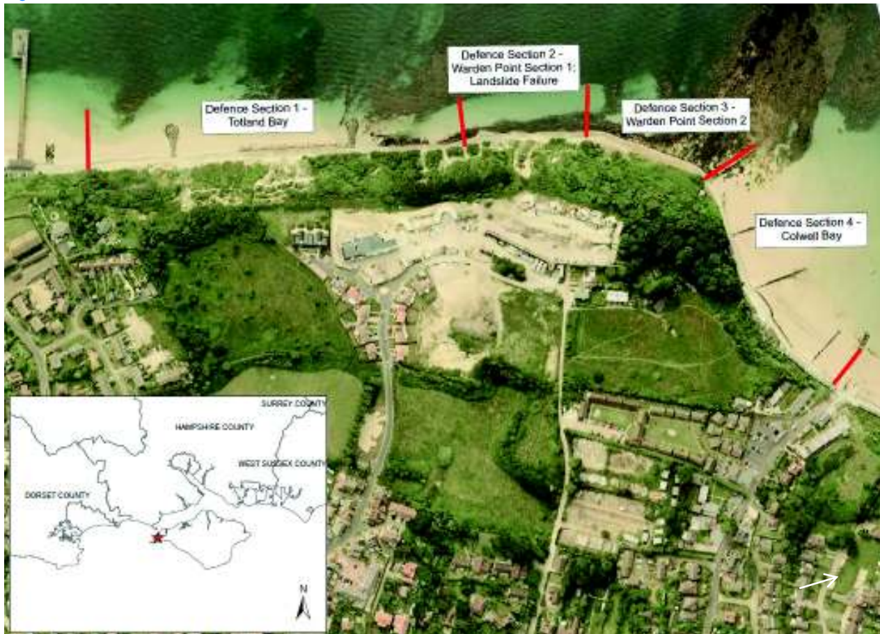
Figure 3.2: The location of the defence sections assessed in the Defence Condition Assessment
