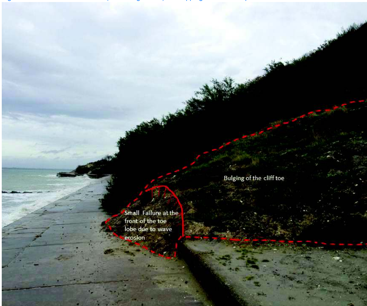
Figure 4.7: Toe of the landslide (seen in figure 4.6) overtopping the concrete promenade
