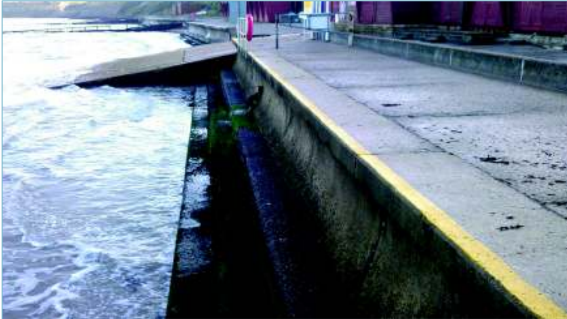
Figure 8.10: Defence Section 4 – Colwell Bay Seawall to Slipway
