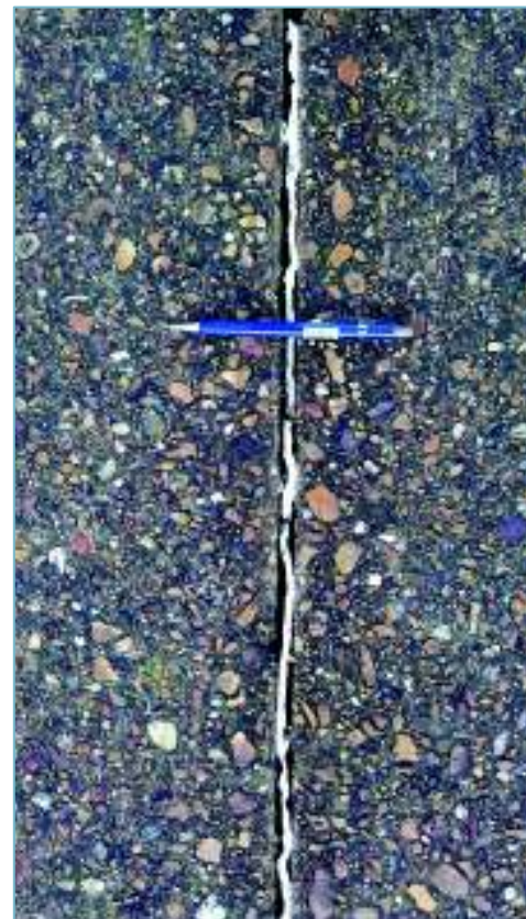
Right: First joint in area of potential movement
