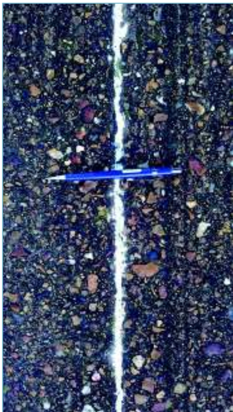
Left: Joint along section without movement,
