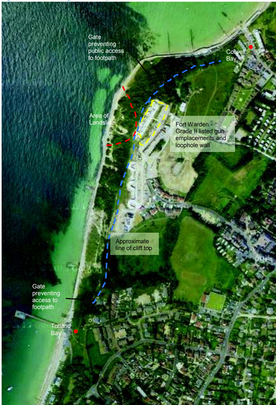
Figure 2.2: Aerial image with the key locations labelled.
