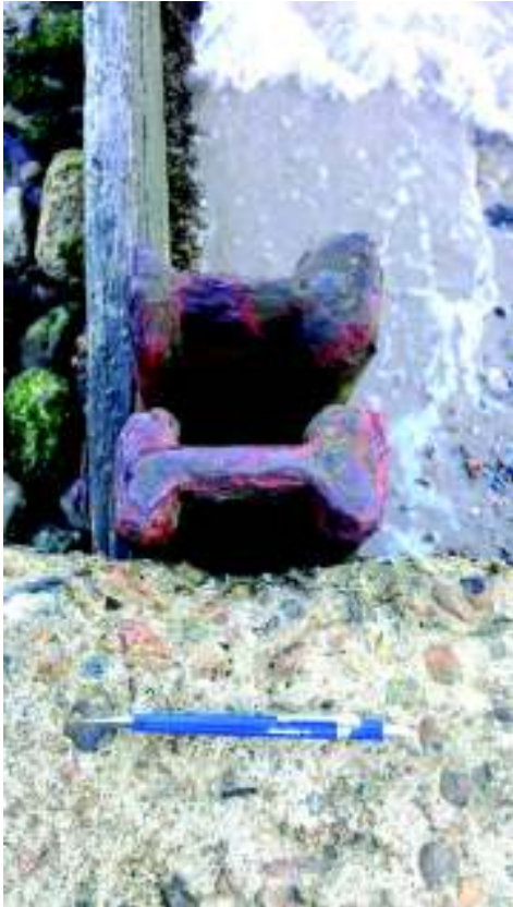
Figure 8.11: Defence Section 4 – Timber groynes straight and example “I” piles
