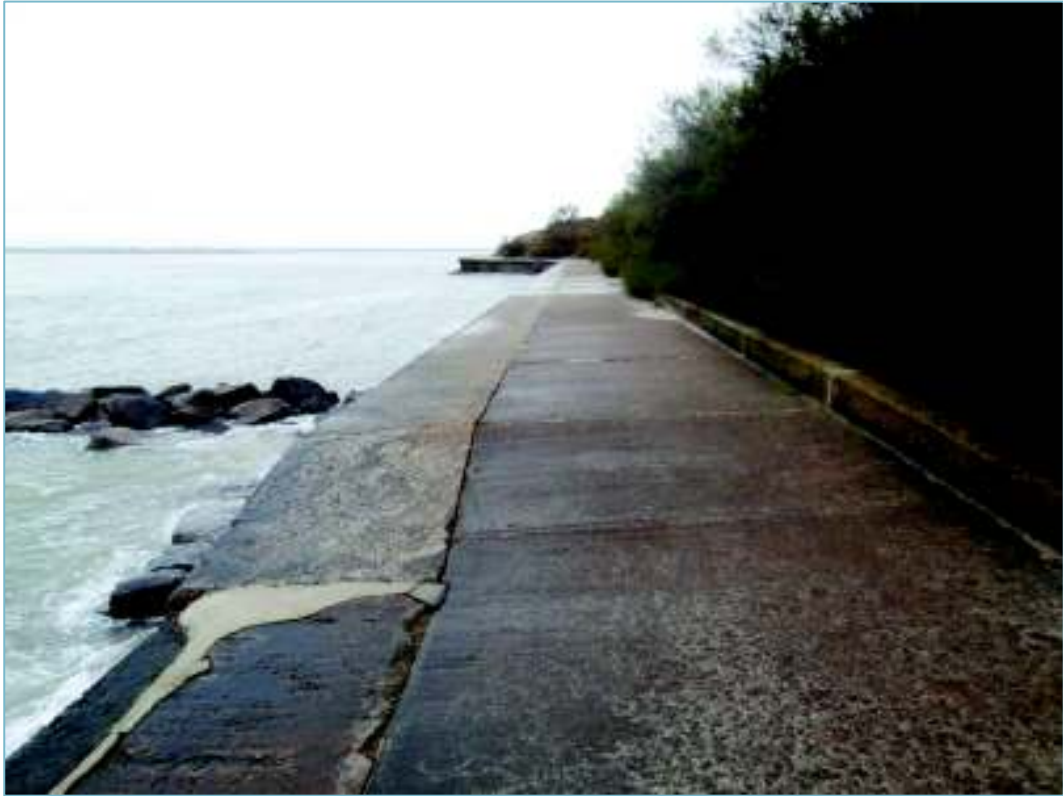
Figure 8.3: Defence Section 1 North – No current signs of seawall movement
