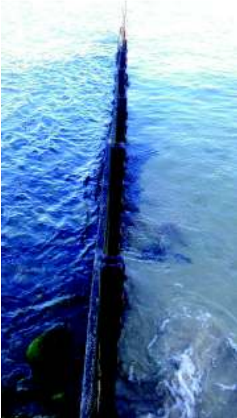
Figure 8.11: Defence Section 4 – Timber groynes straight and example “I” piles
