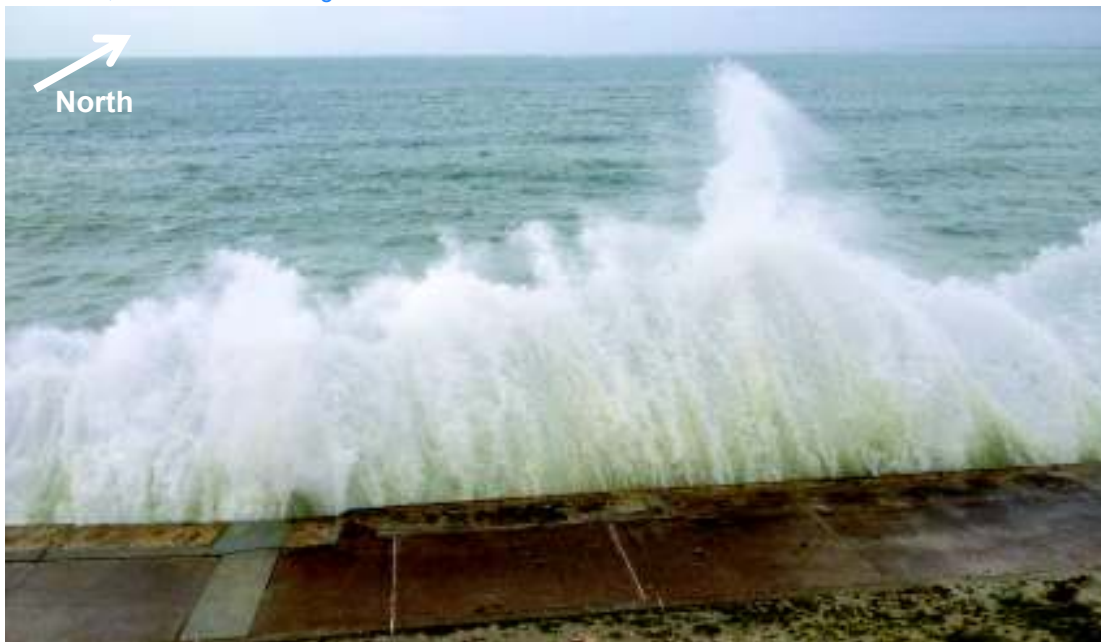
Figure 5.3: Waves overtopping the seawall on 22 nd October 2013. Photo taken along the frontage south of the Landslide, from the cliff looking NW.
