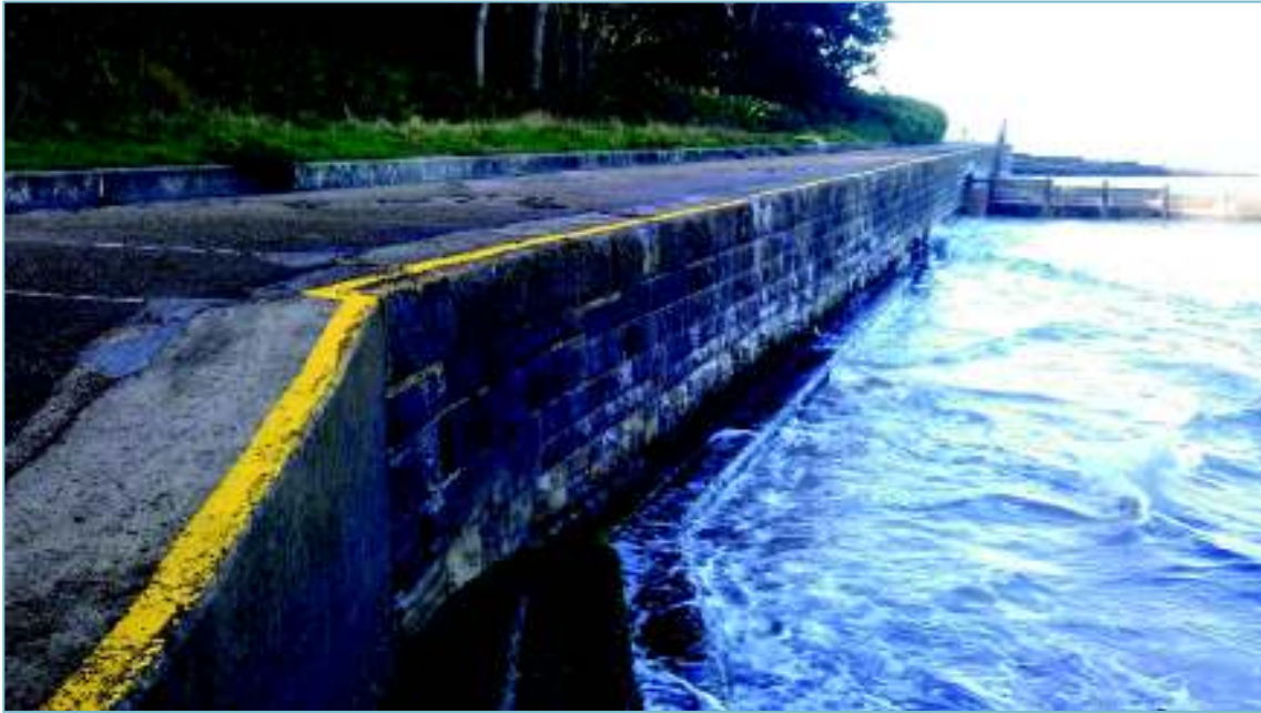
Figure 8.8: Defence Section 4 – Masonry Seawall north of Warden Point
