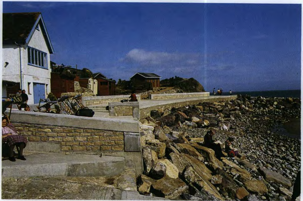
Plate 19. Coastal protection works, Steephill Cove, 1991.
