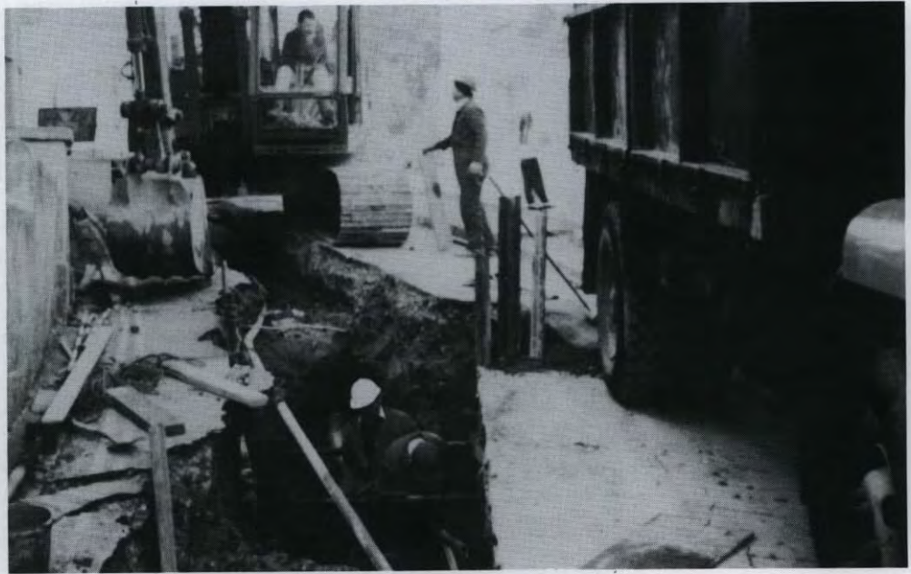
Plate 16. Sewer improvement works, Ventnor Esplanade.
