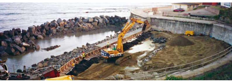
Constructing the new coastal defences seaward of the existing wall in order to provide support for the slope behind.
