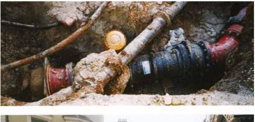
Wherever possible new pipes should be constructed of materials that can accommodate some limited ground movement. This can be assisted by the use of slip joints.
