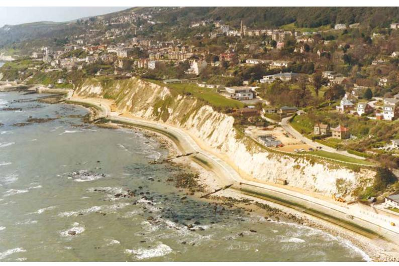
The Bonchurch to Wheeler's Bay coast protection scheme was opened in 1987. Designed for South Wight Borough Council by Lewis and Duvivier, the scheme has eliminated coastal erosion risk for part of Bonchurch as well as assisting in reducing instability.
