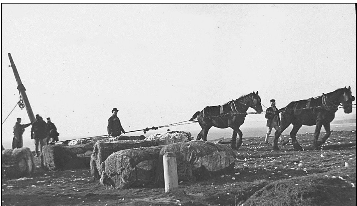
Eider. A team of cart horses with a hoist are lifting large cotton bales from the Eider to the top of the cliff during salvage operations.
