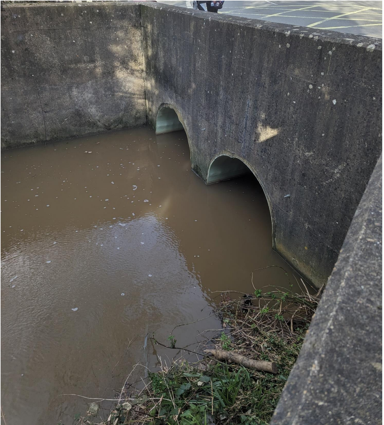
Figure 8-10 Upstream headwall and twin culvert along the watercourse
