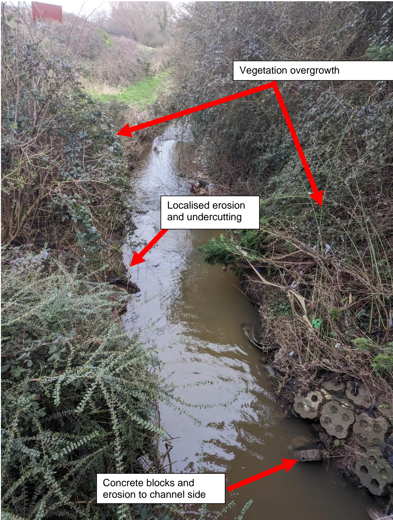
Figure 8-4 Watercourse looking downstream from the Gunville Road highway bridge, right bank with the concrete blocks
