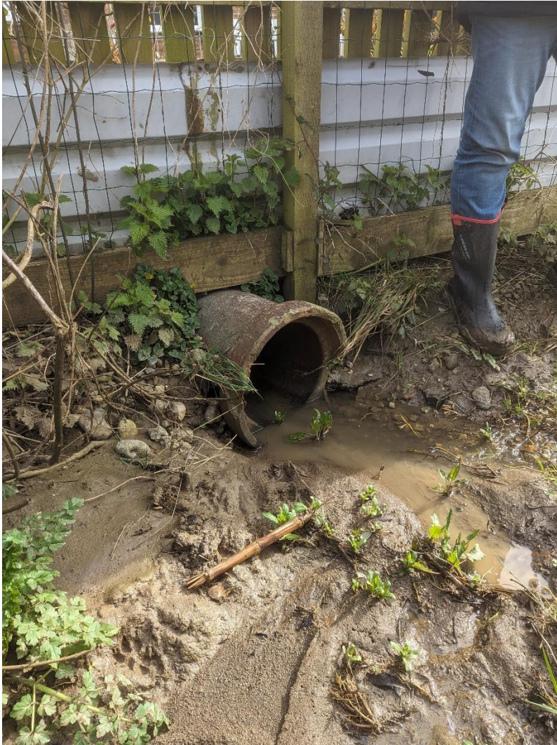
Figure 7-8 Photograph 4, 300mm culvert passing under Arthur Moody Drive, from neighbouring fields
