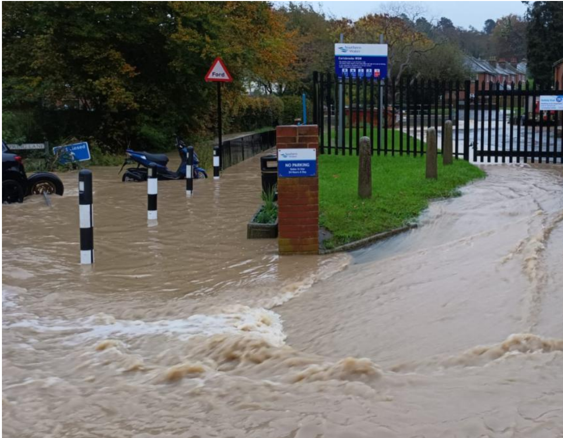
Figure 7-16 Photograph 10, flooding on Spring Lane, looking southeast
