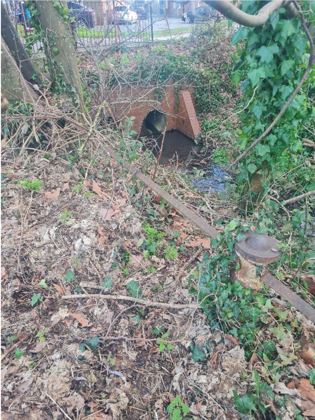
Figure 7-17 Photograph of twin culvert on the ordinary watercourse at Mill Court
