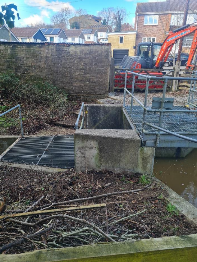
Figure 7-19 Photograph of debris screen on Gunville Stream, near Hunnyhill Aquatics
