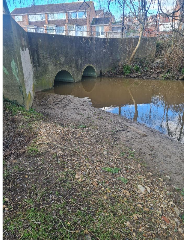
Figure 7-18 Photographs of twin culvert on Gunville Stream, at Towngate Pond
