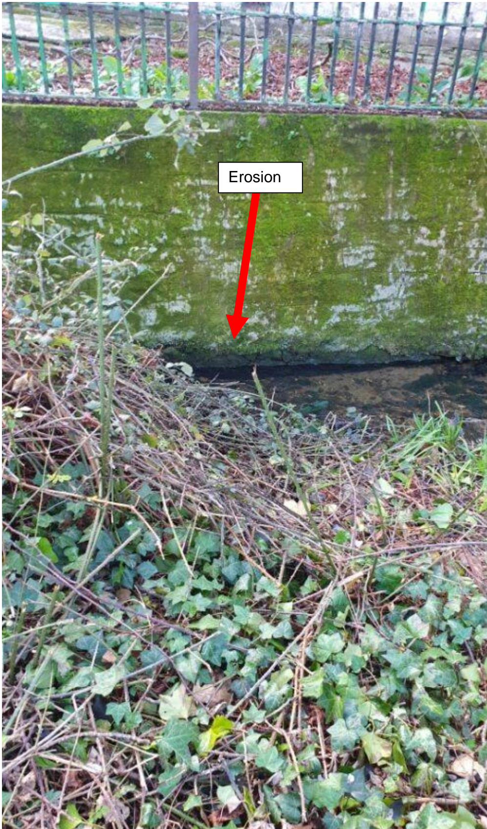
Figure 9-6 Wall, looking south from the right bank
