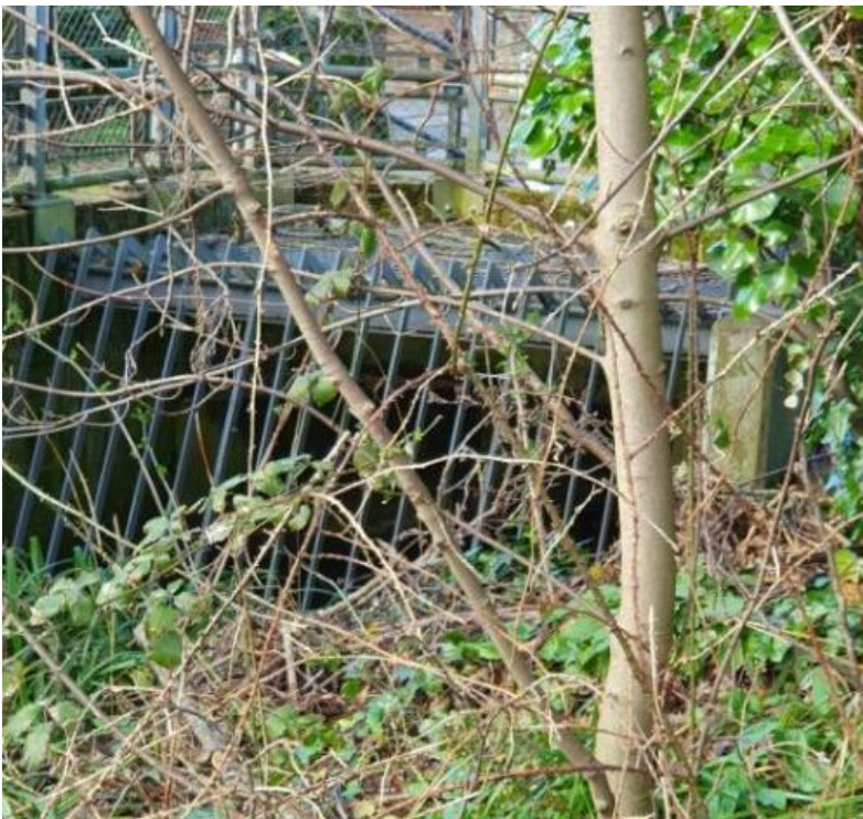
Figure 9-1 Simple culvert, looking northwest from further down on the right bank
