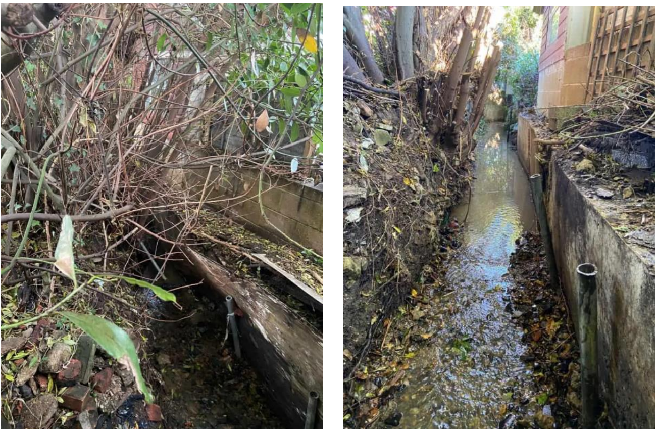
Figure 4-2: Photograph showing watercourse flowing through gardens on Cemetery Road.
