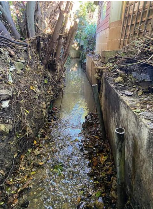
Figure 5-2: The watercourse after the removal of vegetation and debris
