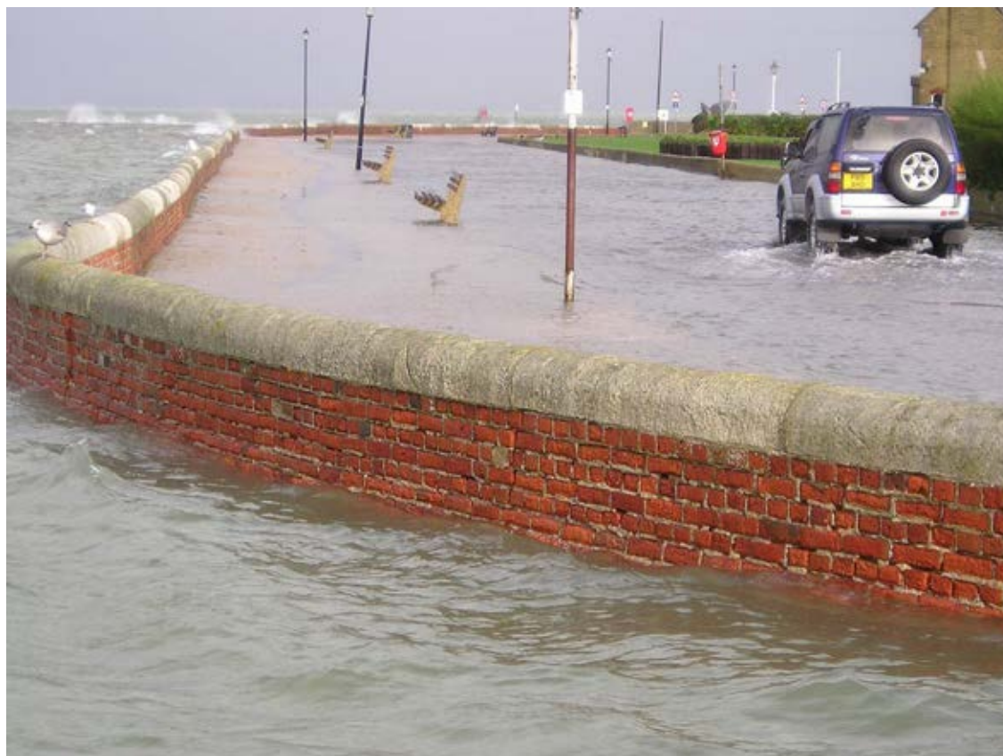
Plate 4: Breach of sea wall at East Cowes (source: Isle of Wight Council)
