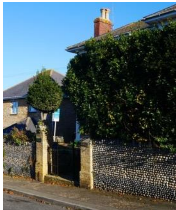
Figure 15 - Local flint walls to a residential property with a hint of grandeur with stone piers to the entrance.
