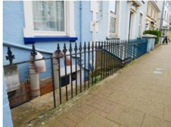
Figure 13 - Minimal repairs to reinstate the continuity of traditional railings.
