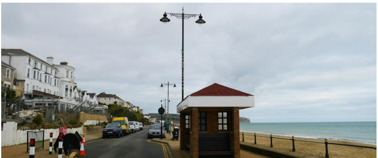
Figure 22 – 23 - A joined-up approach is required to improve the appearance of the Esplanade, its buildings, accessibility and public realm.
