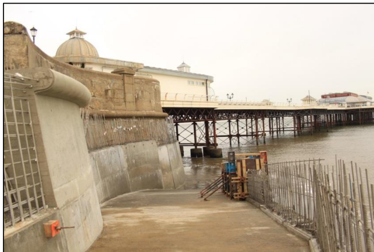
Figure 4-2. Photograph of Cromer seawall encasement
