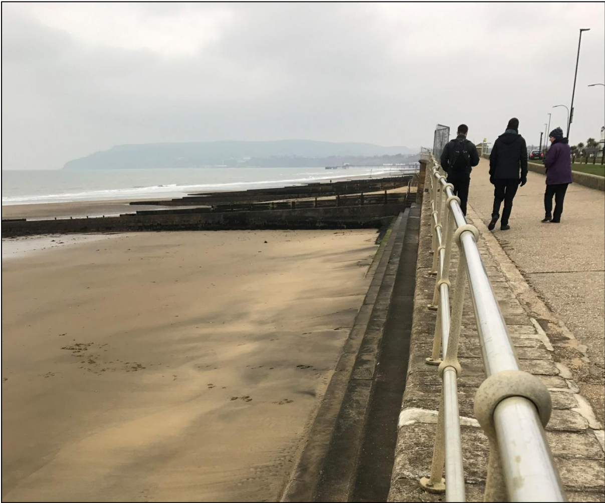
Figure 6-3. Members of the project team inspect the defences in Unit IW23
