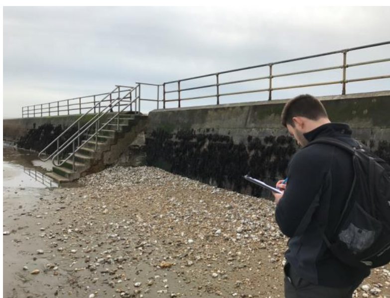
Figure 2-1. AECOM visual asset inspection (March 6 th 2017).
