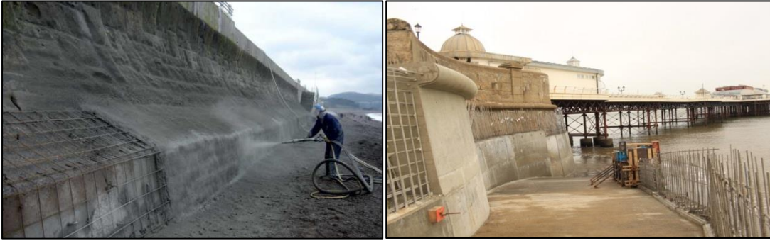
Figure 6-1. Photographs showing examples of concrete spraying of a seawall at Minehead (left) and encasement at Cromer (right)
