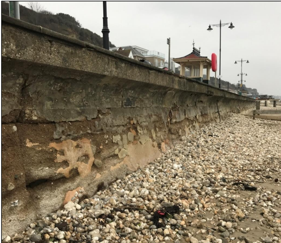
Figure 6-7. IW27 seawall in poor condition (southern end of the esplanade)
