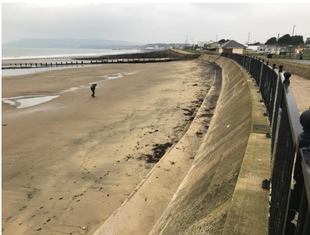
Figure 4-1. Seawall between Sandown Zoo and Culver Parade
