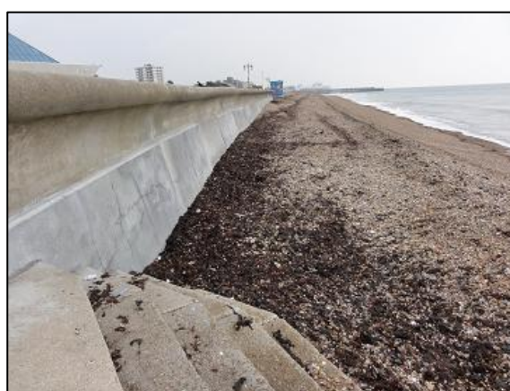
Figure 4-3. Example of crest raising at the top of the defence (left, Sandown) and a wave return wall (right, Pevensy)
