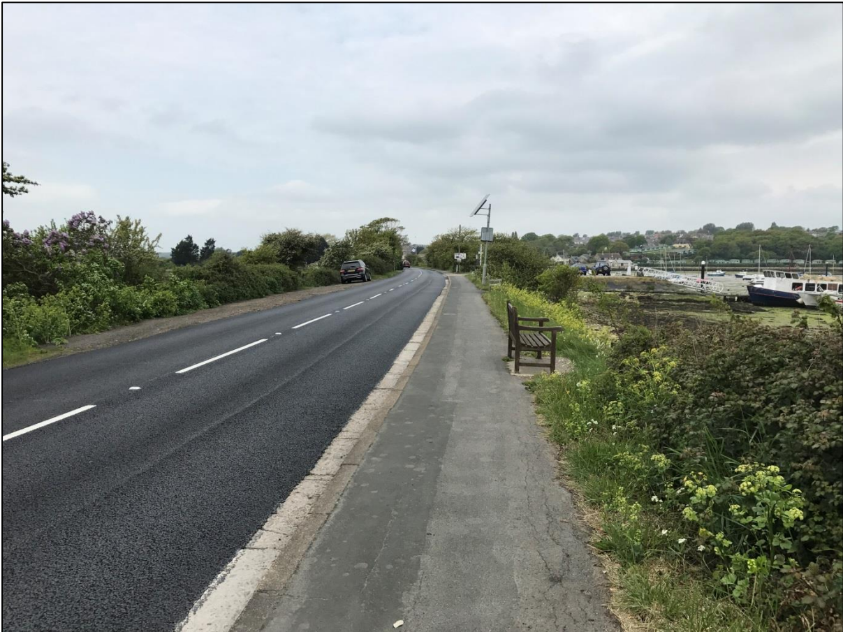
Figure 6-10. Embankment Road (looking west)
