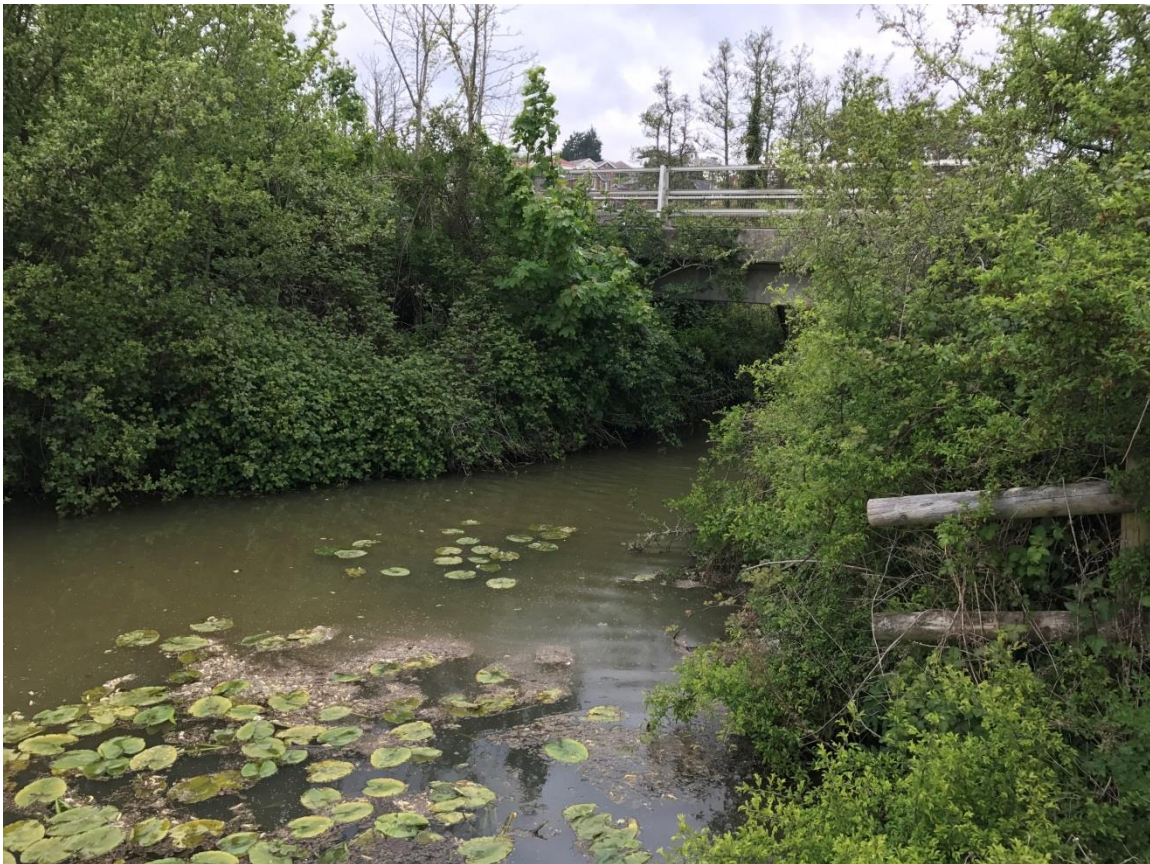
Figure 7-5. Photograph of the bridge crossing across the Eastern Yar at Yarbridge. Photograph looking north.
