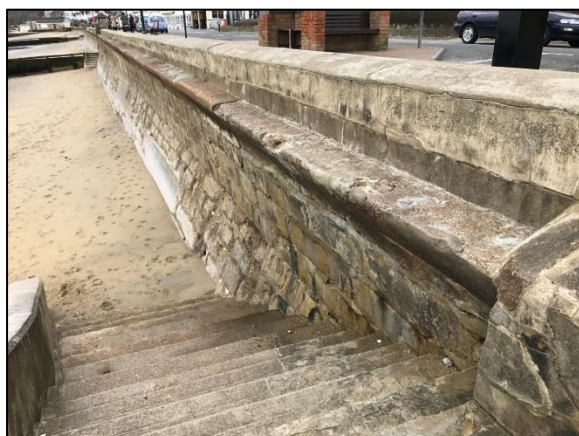
Figure 4-3. Example of crest raising at the top of the defence (left, Sandown) and a wave return wall (right, Pevensy)
