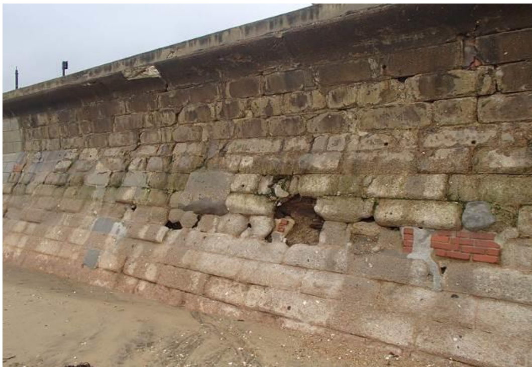
Figure 4-4. Photograph showing the seawall at North Shanklin (IW27 002).
