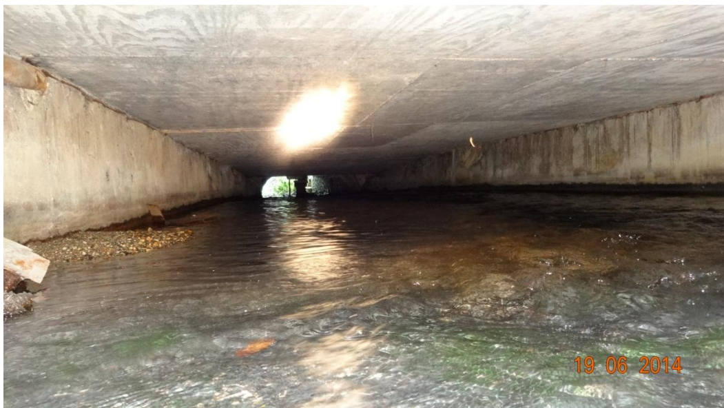
Figure 4: Cedar Hill Culvert
