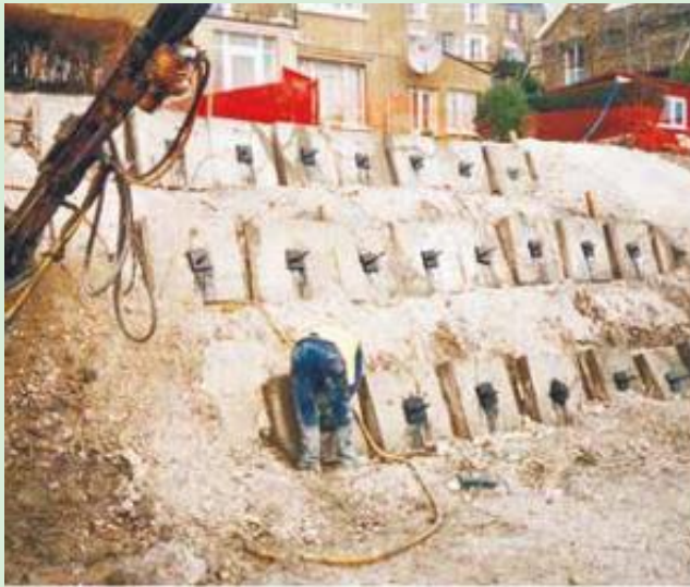
Soil nailing the upper slope
