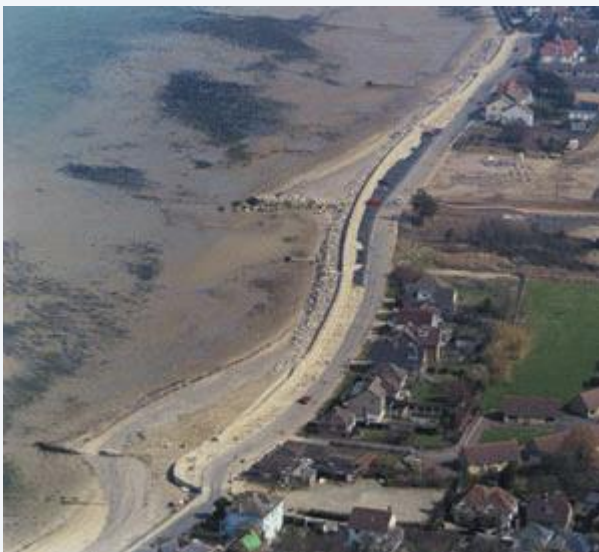
The Completed Seaview Duver Scheme
