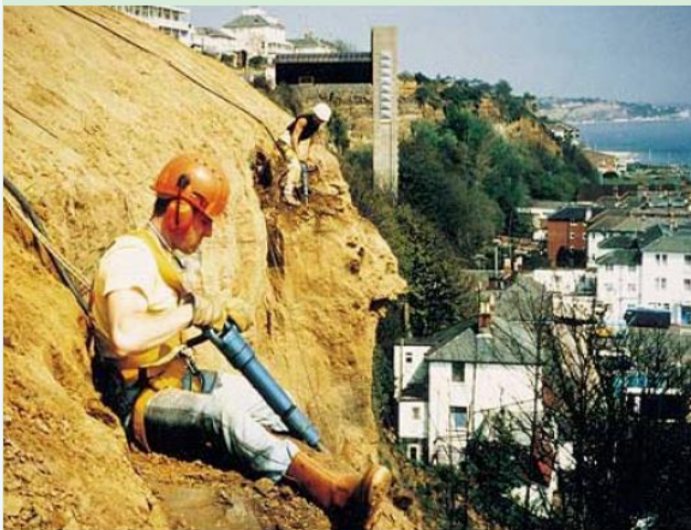
Past cliff stabilisation works in Shanklin.
