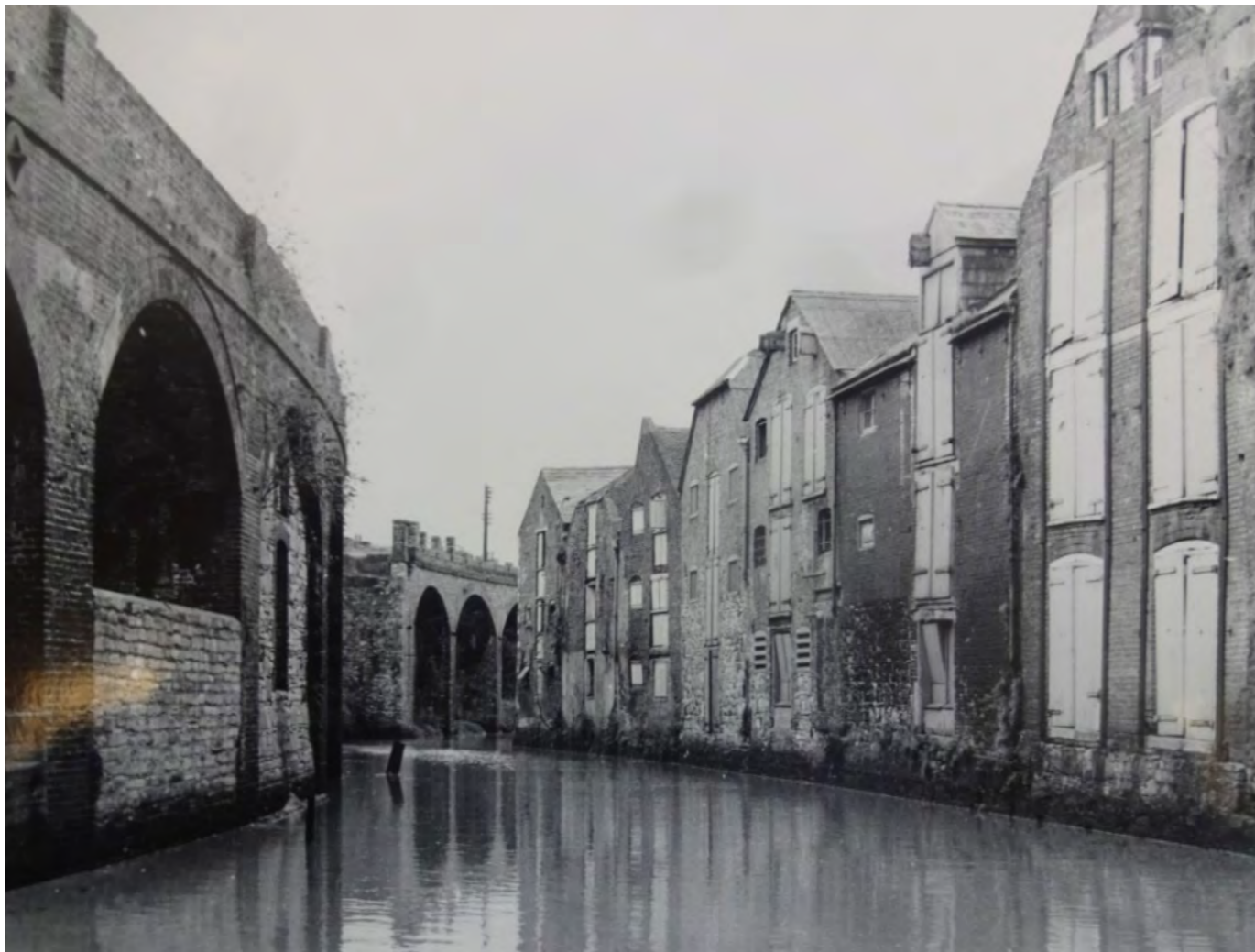
Figure 20. 1970s view of the demolished Sea Street warehouses, from Newport Harbour Historic Area Assessment.
