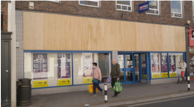
A poor example of an excessive fascia in Newport where the fascia makes up about 50 per cent of the entire shopfront. This makes the shop look like a billboard rather than a commercial premises.
