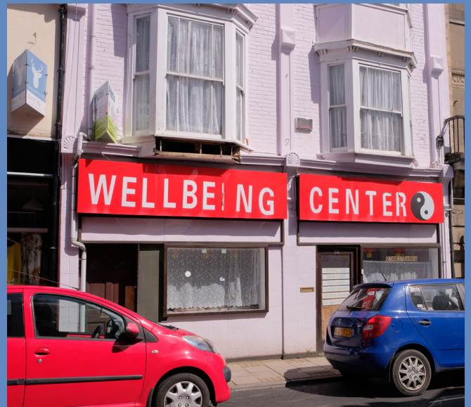
Existing shopfront 51-52 High Street
