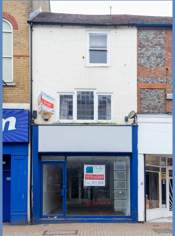
Existing shopfront 59 High Street
