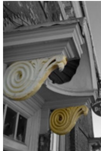
Examples of ornate console brackets in Newport and Ryde.
