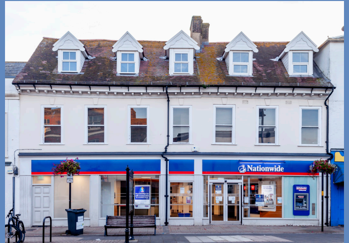
Existing shopfront 22 St James' Square
