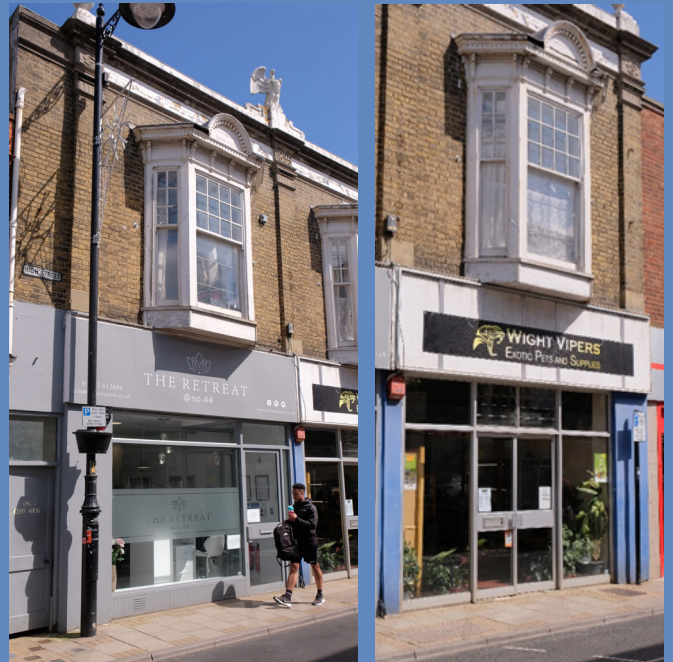
Existing shopfronts 44-45 High Street
