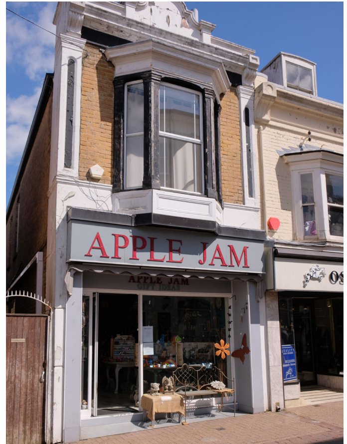
The engaged pilasters on this shop's upper storey would once have once framed the entire façade
