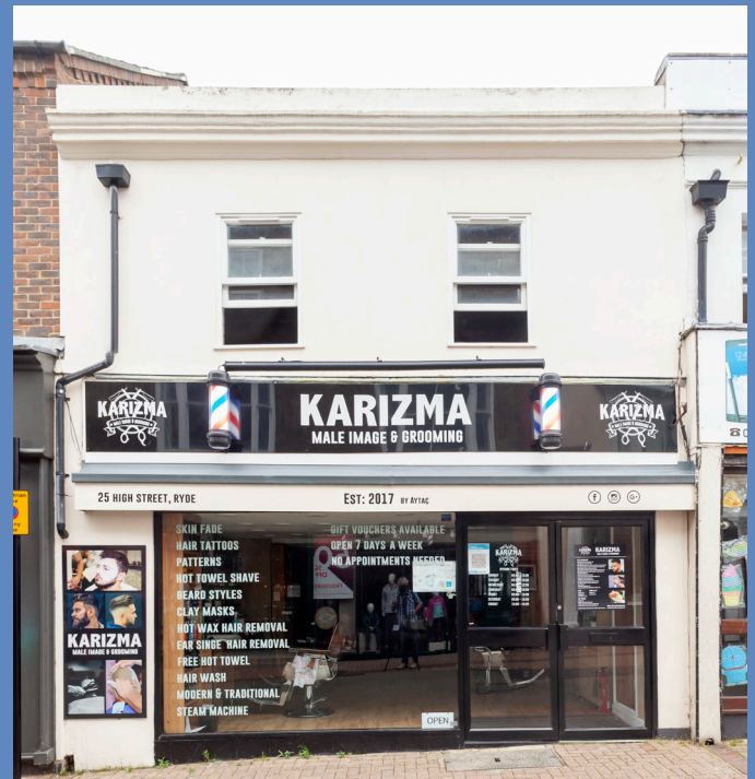
Existing shopfront 25 High Street
