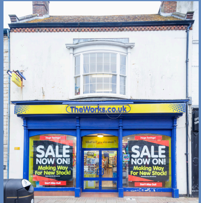
Existing shopfront 19 St James' Square
