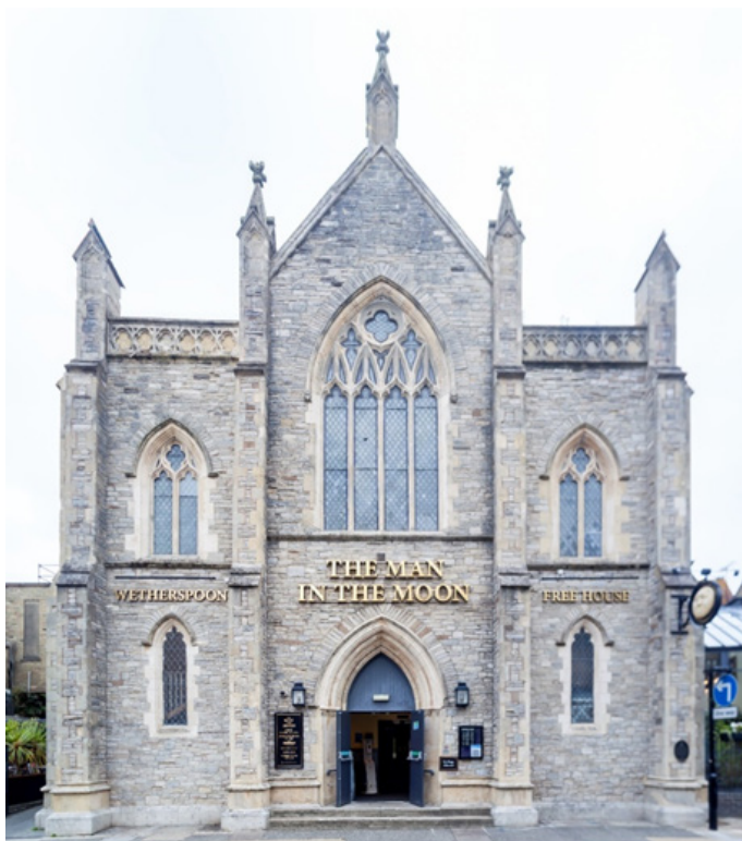
The Man in the Moon is one of the most popular examples of a (now) commercial frontages in Newport according to the survey undertaken in support of this guidance. It reuses the frontage of the former Congregational Church with minimal additions.
