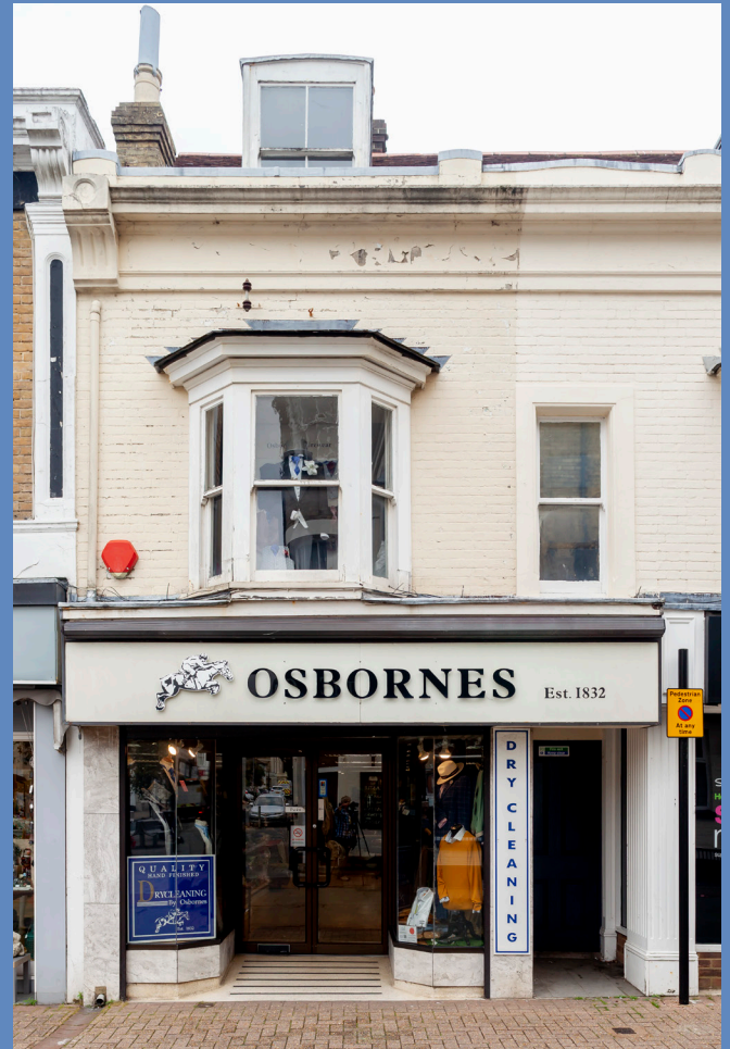
Existing shopfront 29 High Street
