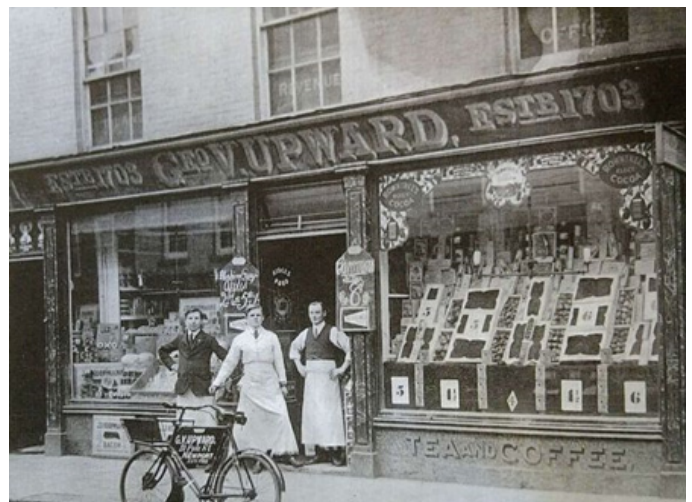
Historic archive photographs show the use of the largest possible letters when sign writing. Newport. Note the signwriting on the stall riser also.
