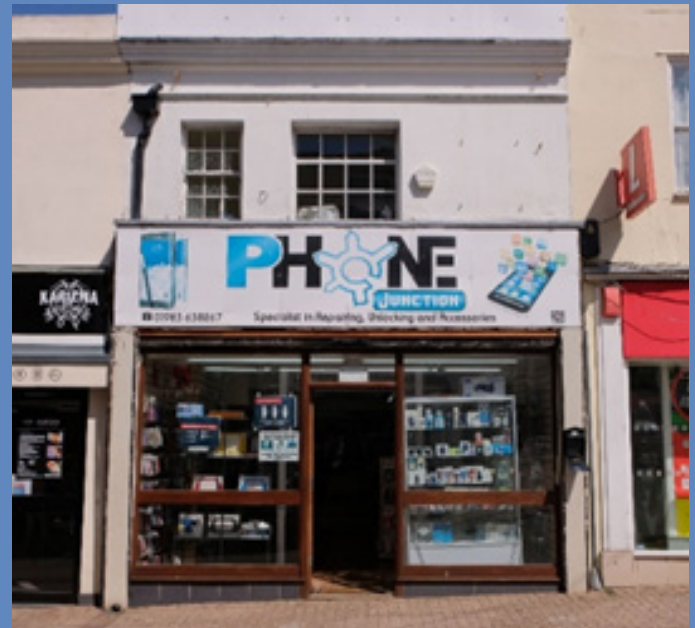
Existing shopfront 26 High Street
