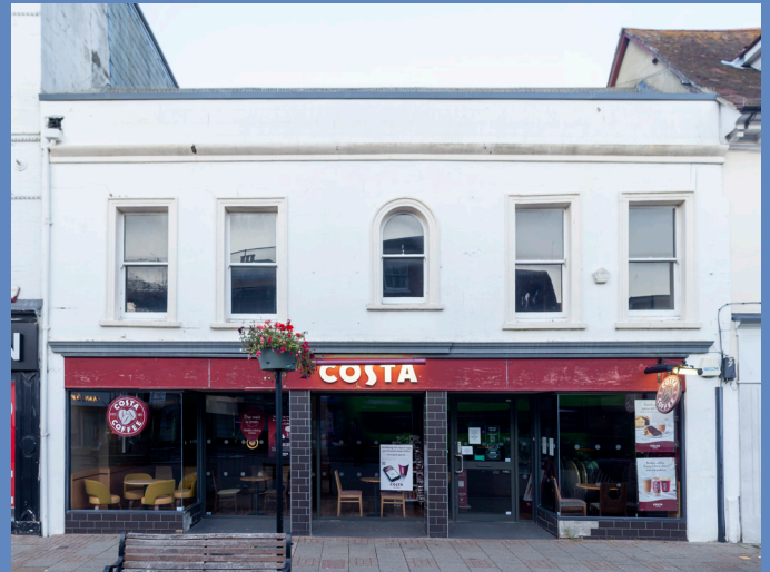
Existing shopfront 21 St James' Square
