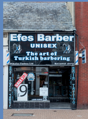
Existing shopfronts 92-94 High Street
