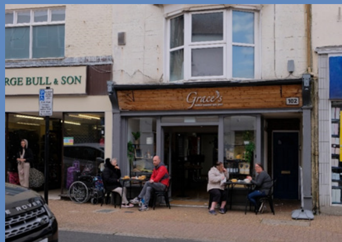
Existing shopfront 101 High Street
