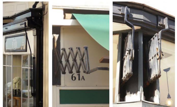
Existing blinds, Ryde
