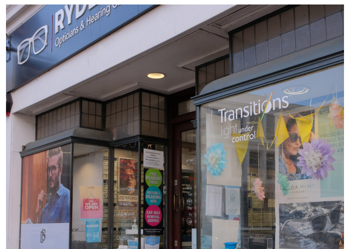
Increasing the opacity of transom lights allows false ceilings to be concealed without compromising the appearance of the shopfront
