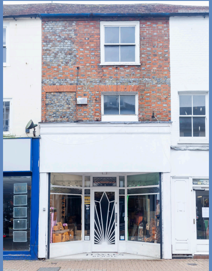
Existing shopfront 60 High Street
