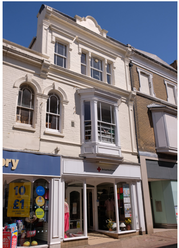
Shopfront improvements should be considered within the context of the whole building.
