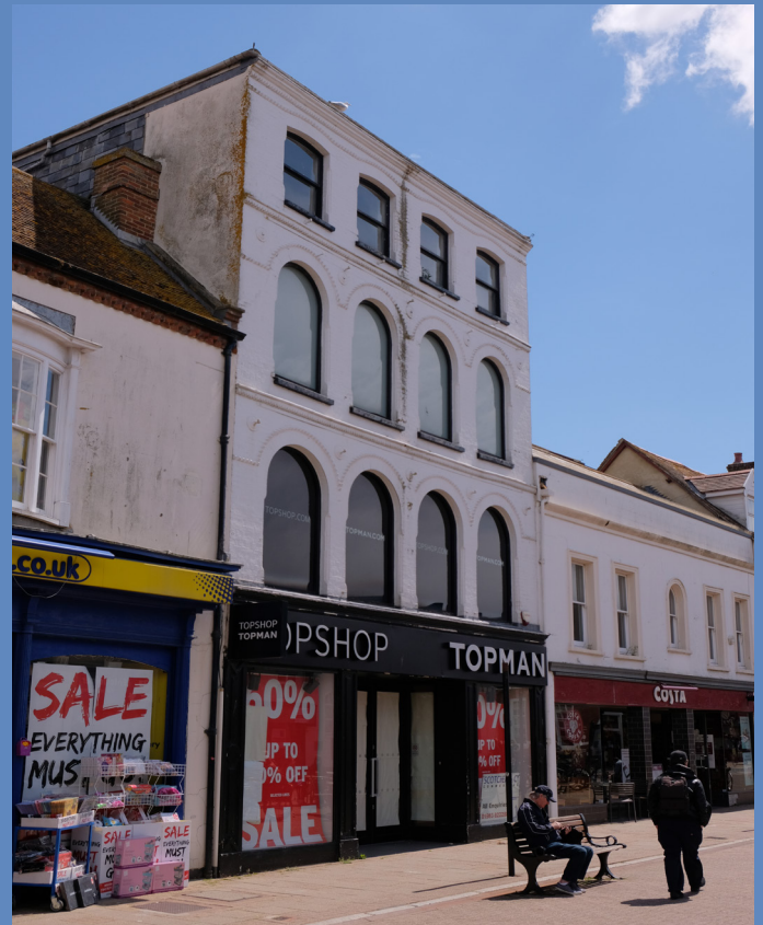
Existing shopfront 20 St James' Square
