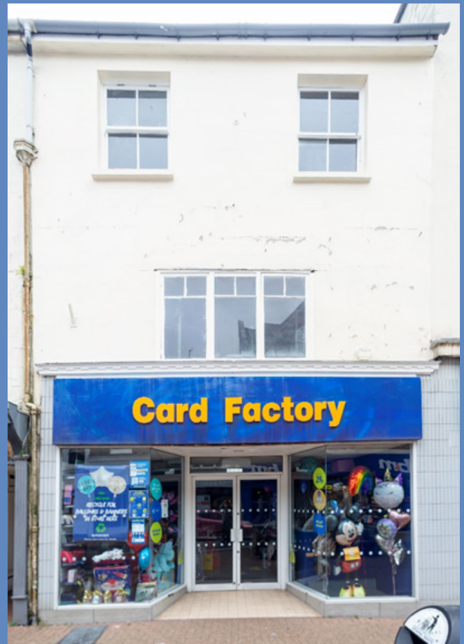
Existing shopfront 103 High Street
