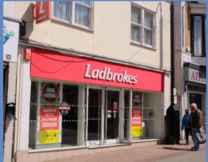
Existing shopfront 27 High Street
