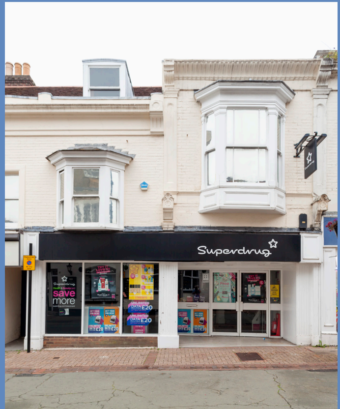
Existing shopfront 30-31 High Street
