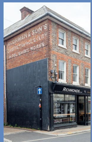
Existing painted sign on the side of a nearby building in St James' Square, Newport
