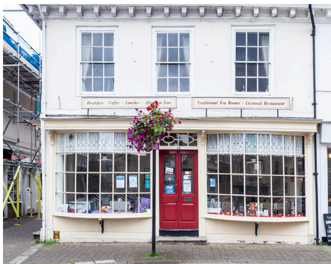
An example of a Georgian ground-floor bow window, God's Providence House, Newport
