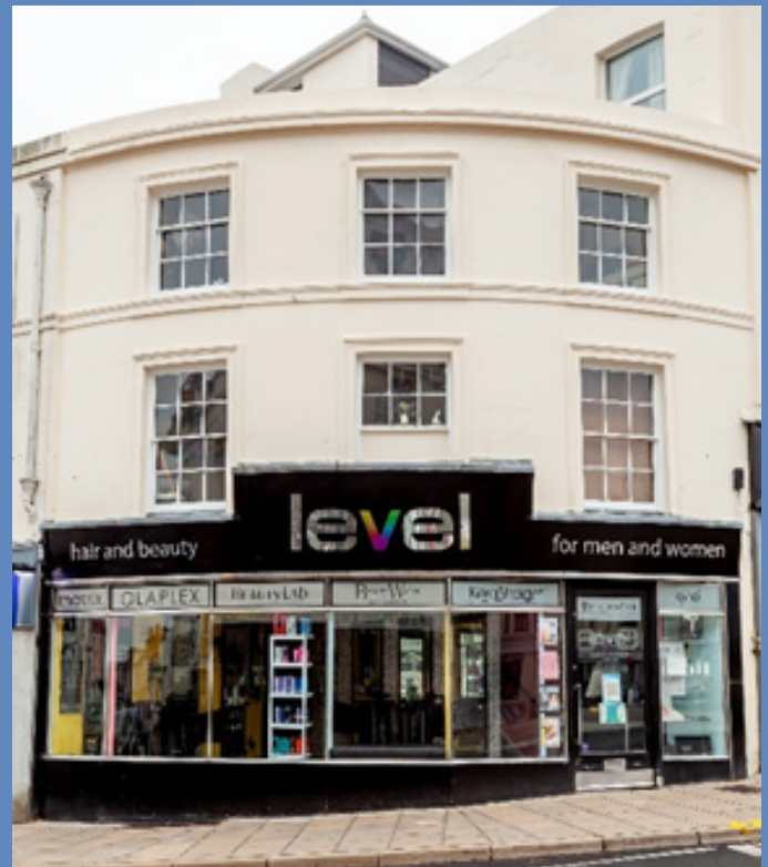
Existing shopfront 4 St Thomas' Square
