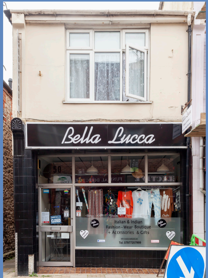
Existing shopfront 50 High Street
