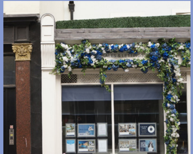
An example of excessive greenery that obscures the view of the fascia
