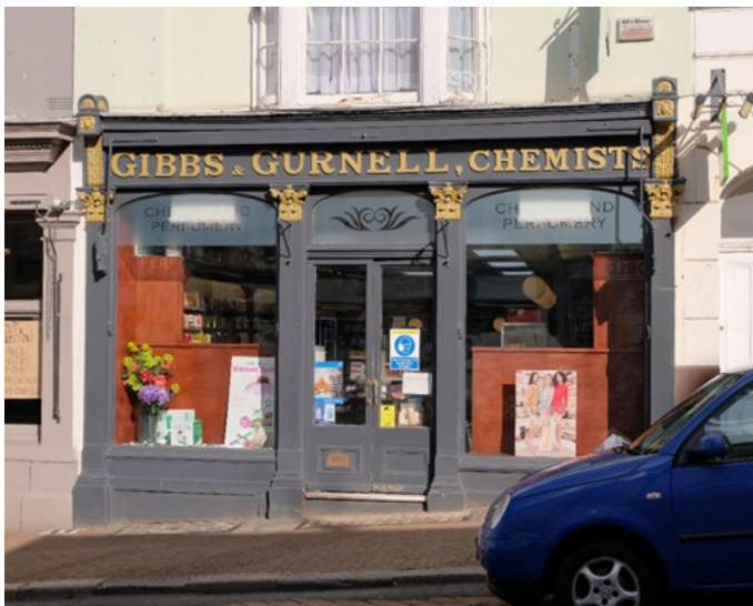
A Victorian shopfront in Ryde
