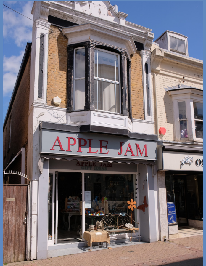
Existing shopfront 28 High Street
