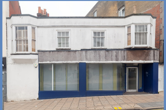
Existing shopfront 9 St Thomas' Square
