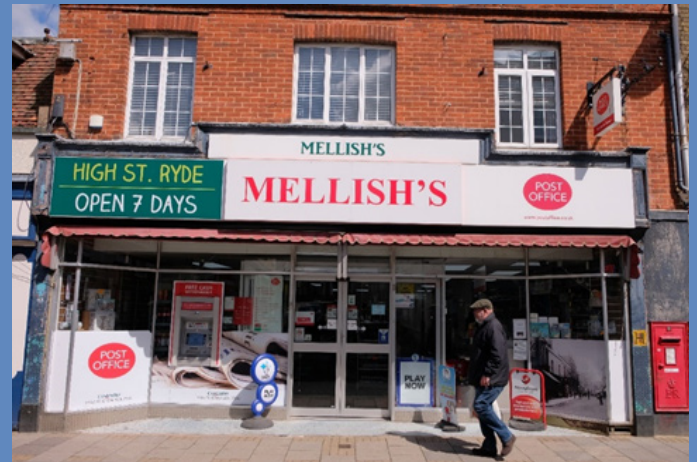
Existing shopfront 43 High Street
