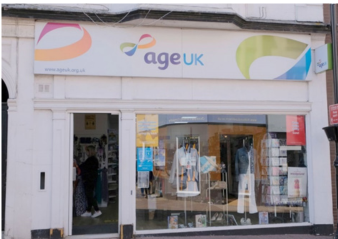
A poor example of a modern fascia mounted on, and obscuring architectural detail of heritage value.
