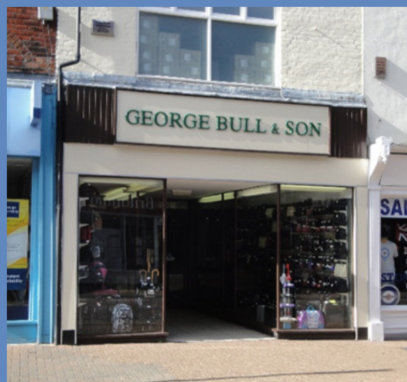
Existing shopfront 101 High Street
