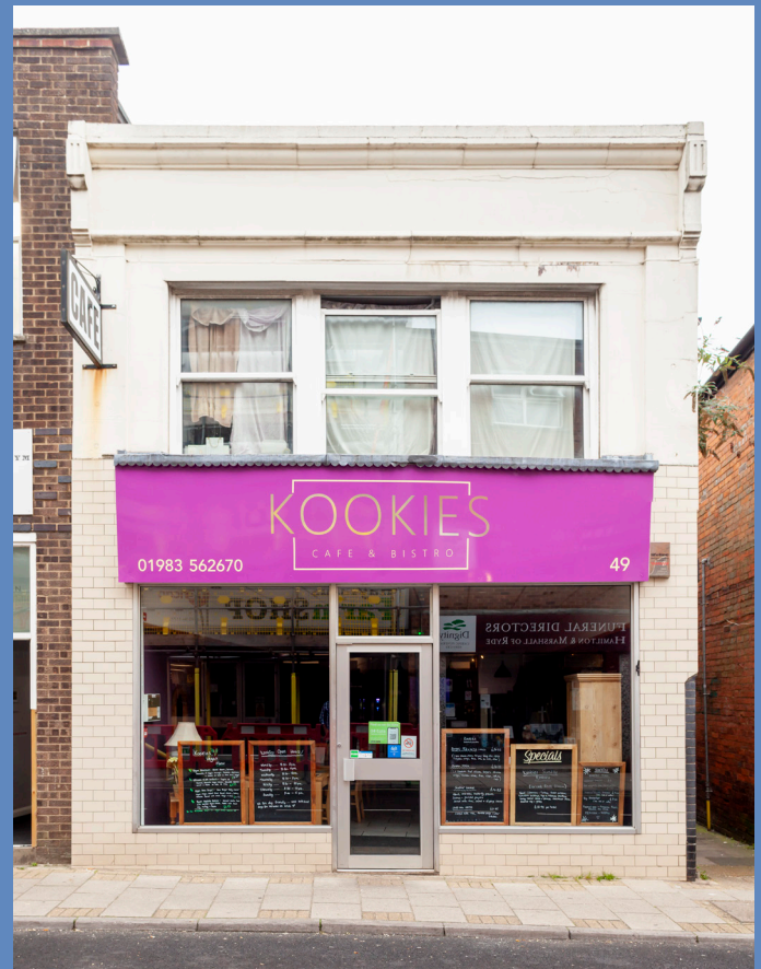
Existing shopfront 49 High Street
