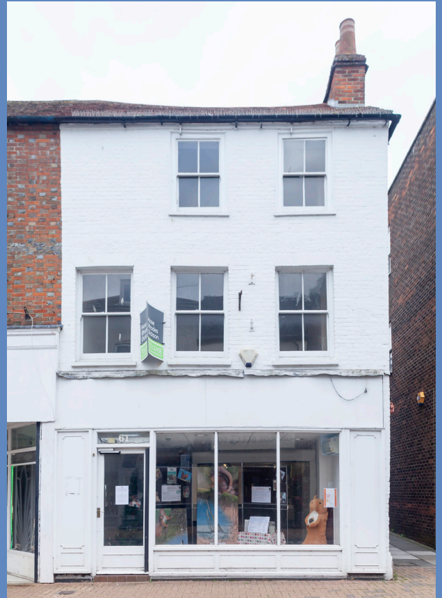
Existing shopfront 61 High Street
