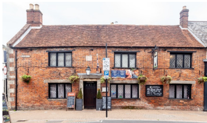
A non-standard commercial frontage in a 17th century building, The Castle Inn, Newport
