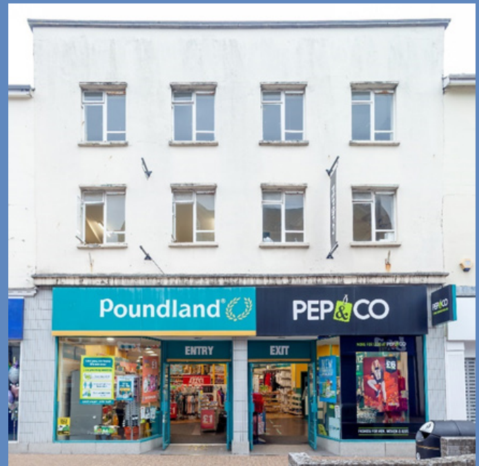
Existing shopfront 104 High Street
