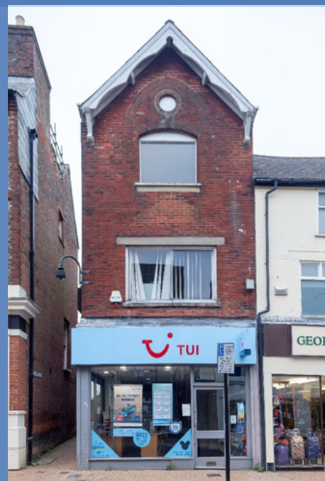
Existing shopfront 100 High Street
