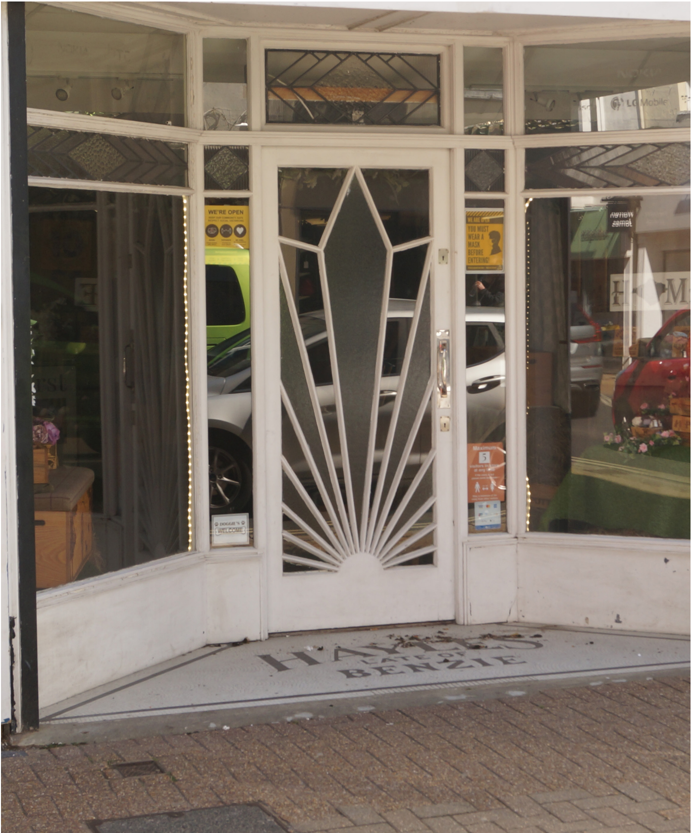
View of the existing art deco shopfront in Hub 2, Newport
