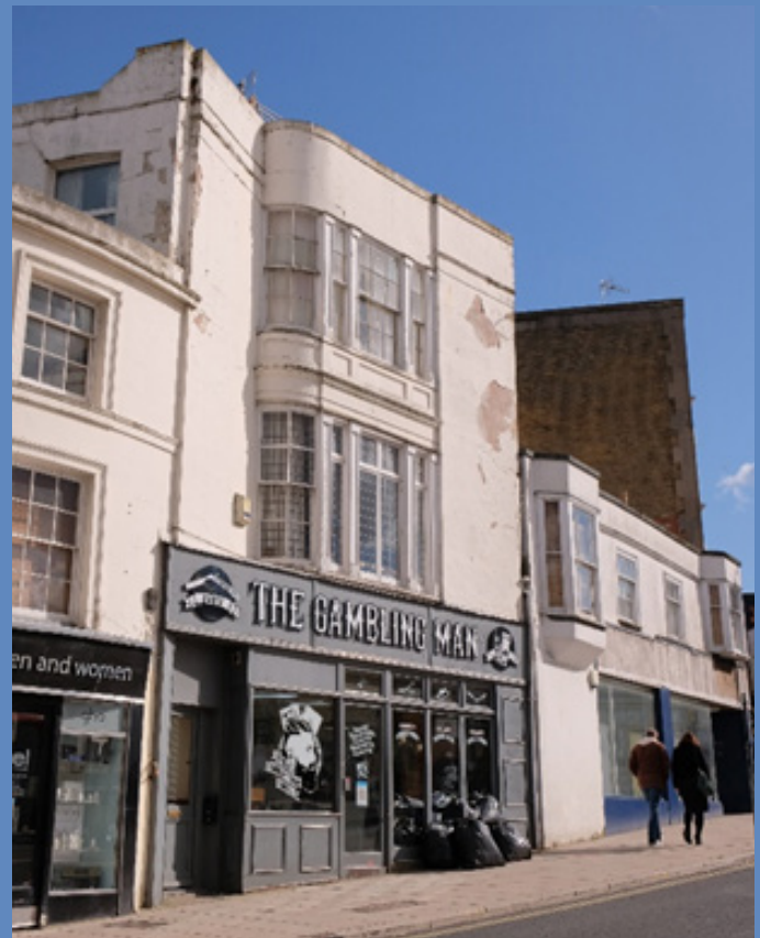
Existing shopfront 5 St Thomas' Square
