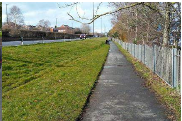
Footpath alongside Medina Way approaching the Isle of Wight College
