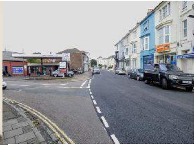
Junction of Monkton Street and East Street
