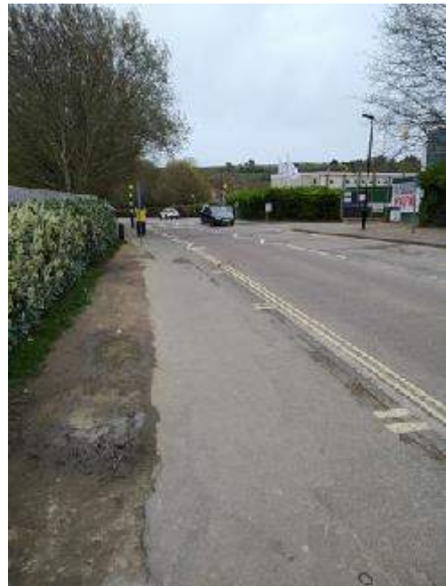
Wellington Road, looking east
