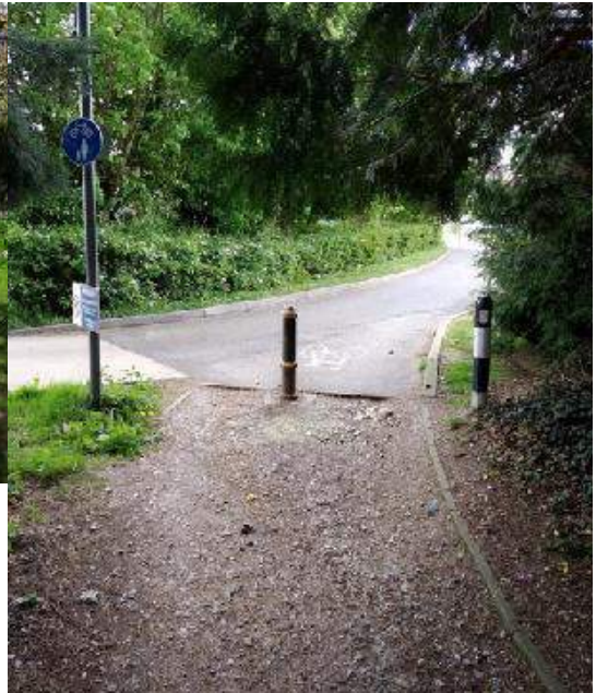
Shared use route south of Medina Leisure Centre
