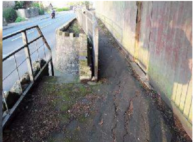
Binstead Road, looking north
