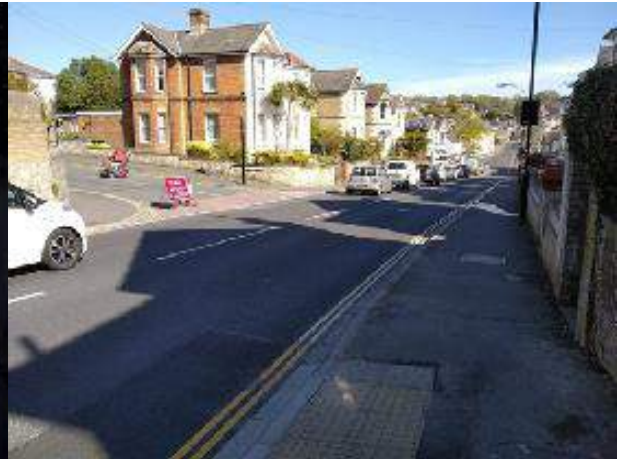
Junction of St Johns Hill and Bennet Street
