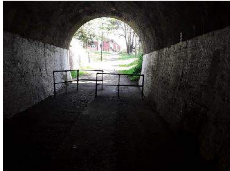
Tunnel under Fairlee Road
