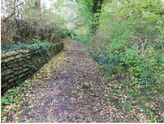
Former rail line parallel to Fairlee Road
