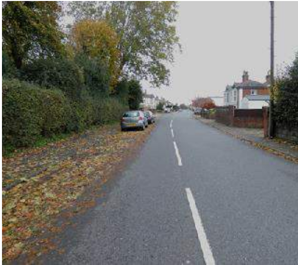
Marlborough Road, looking north
