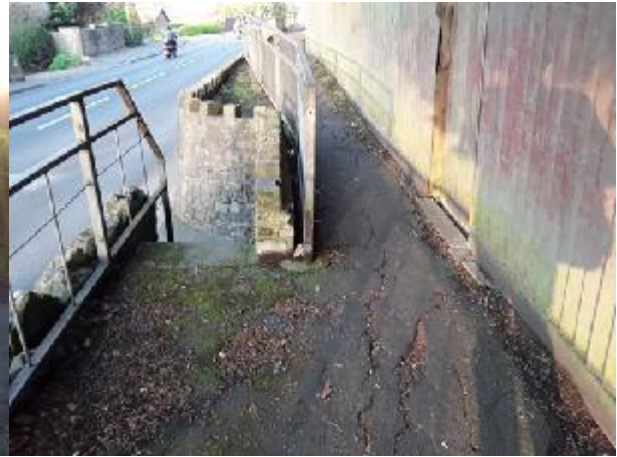
Binstead Road, looking north
