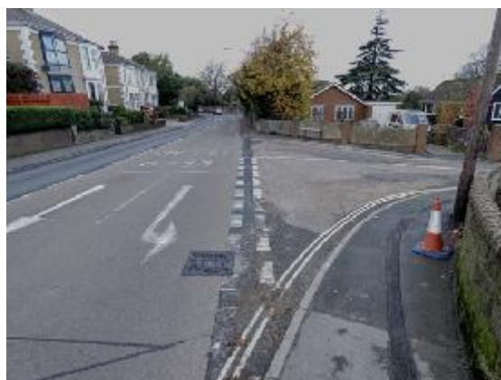
Junction of Binstead Road and Thornbrough Close
