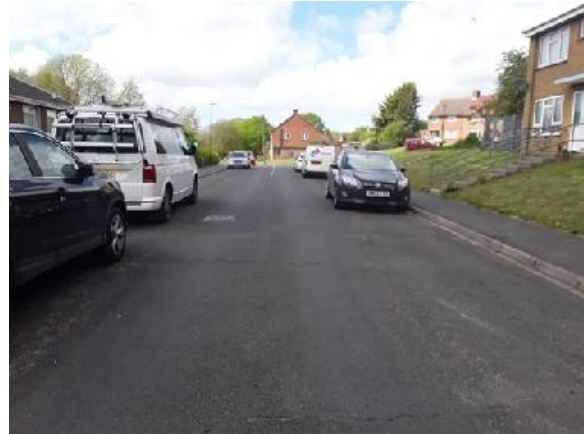
Looking west along Garden Way
