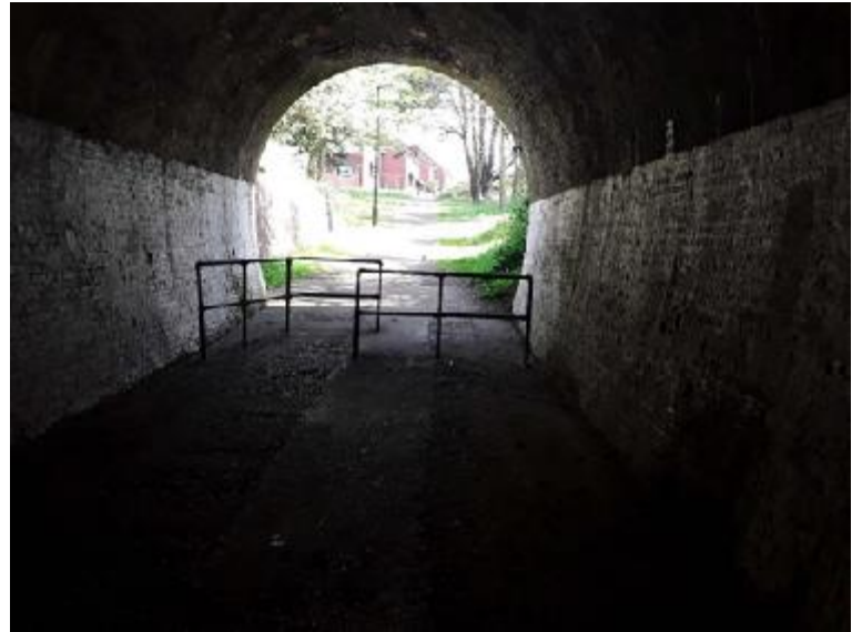
Tunnel under Fairlee Road
