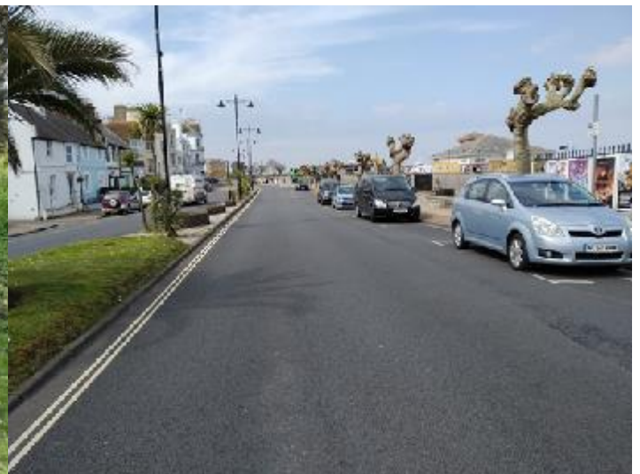
Ryde Esplanade, looking west
