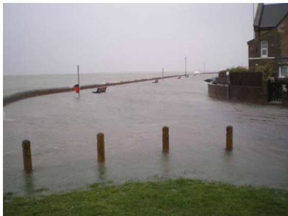
Flooding in East Cowes
