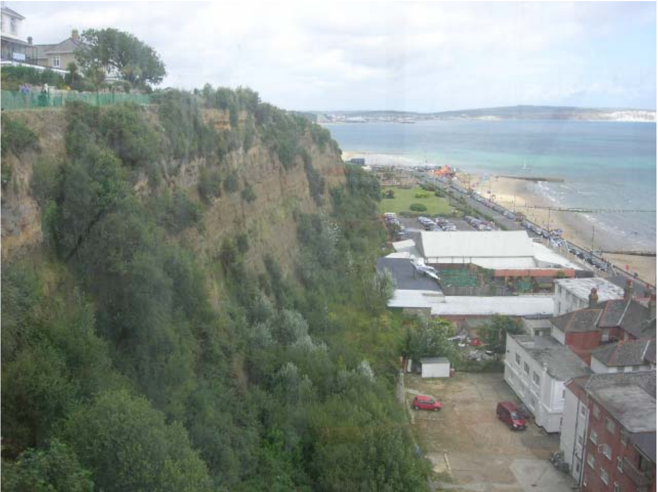
Plate 10: Shanklin Esplanade, showing the former sea cliffs which are subject to rockfall and talus slope failure, with the stabilised built up sediments forming Shanklin Esplanade below, in July 2009.
