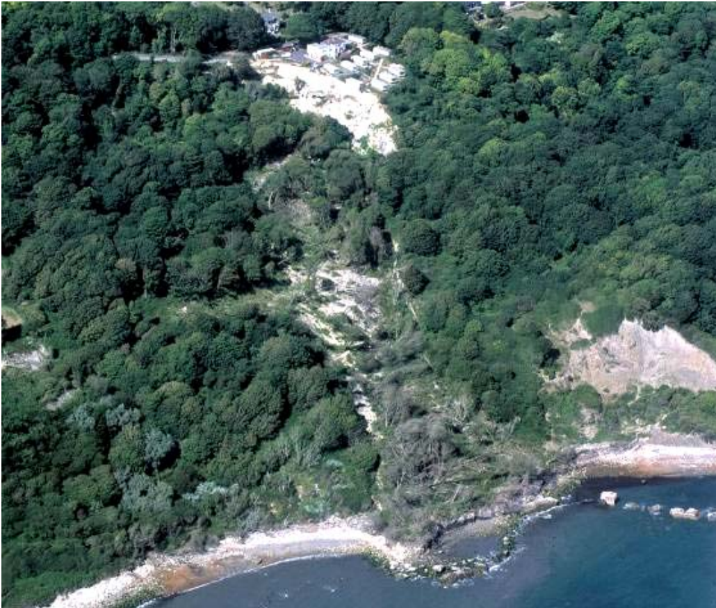
Plate 14: Landslide reactivation along the Niton Undercliff, following prolonged winter rainfall in 2000/2001, affecting the coastal road and a caravan park (Isle of Wight Council).
