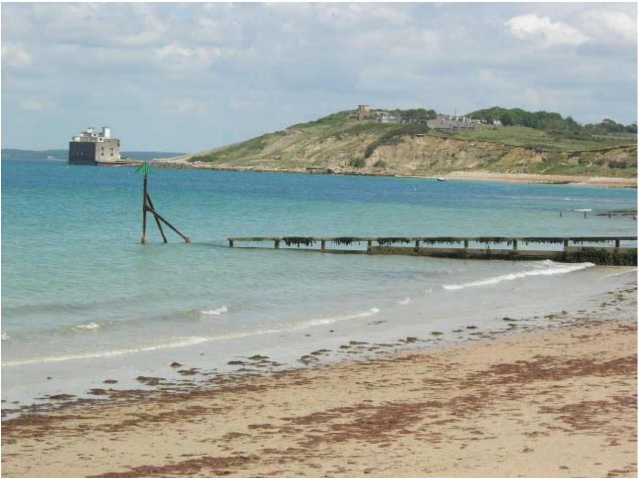
Plate 25: Eroding coastal cliffs in the north of Colwell Bay. View from Colwell Bay (where the south of the bay is defended by a seawall) looking north-east to Fort Albert (Cliff End), June 2009.
