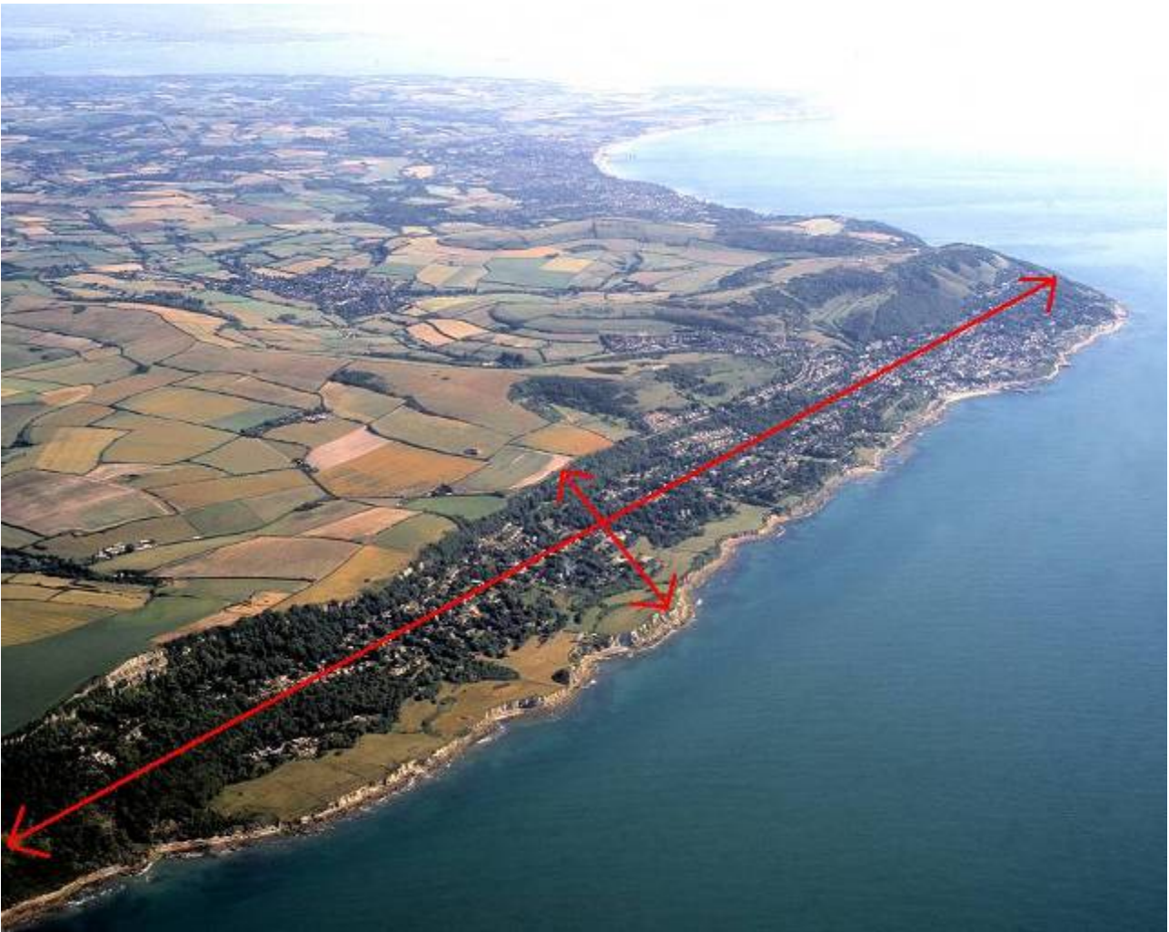
Plate 11: View west along the Ventnor Undercliff Landslide Complex from St. Lawrence to Ventnor. The landslide complex extends 12km along the south coast of the Isle of Wight, from Blackgang to Bonchurch. (Isle of Wight Council).
