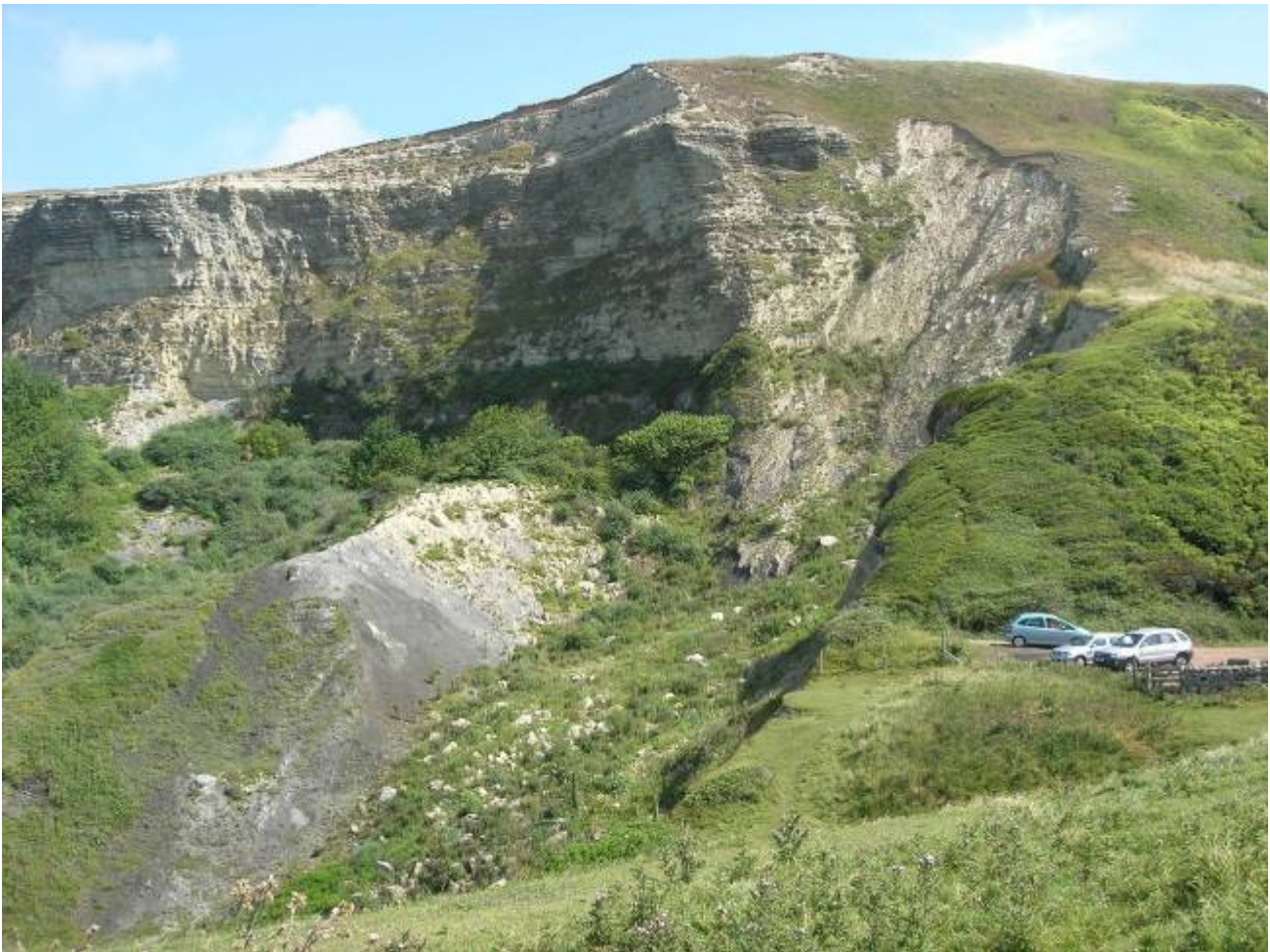
Plate 15: Gore Cliff, with failures from the backscar of the landslide complex and in the Gault Clay and coastal slopes below, near the site of the 1928 Great Cliff Fall which severed the coastal road. July 2006
