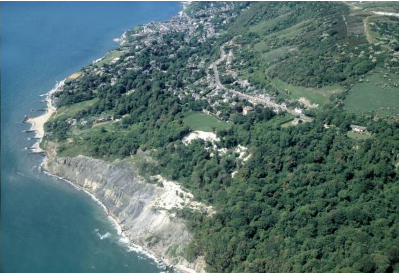
Plate 12: Landsliding and cliff retreat encroaching near the village of Bonchurch (Isle of Wight Council).
