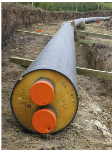
Figure 11 Twin Core Preinsulated Pipe
