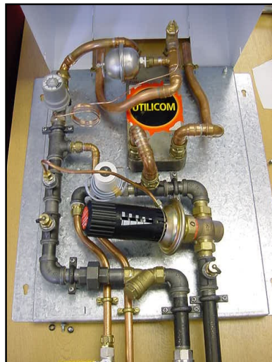
Figure 14 Typical Domestic DH Connection
