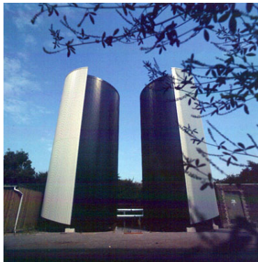
Figure 9 Typical Accumulator Installation
