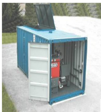
Figure 8 Containerised Biomass Boiler
