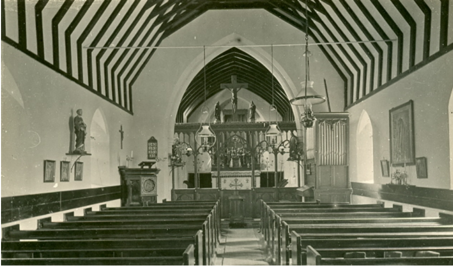
Interior of Havenstreet Parish Church
