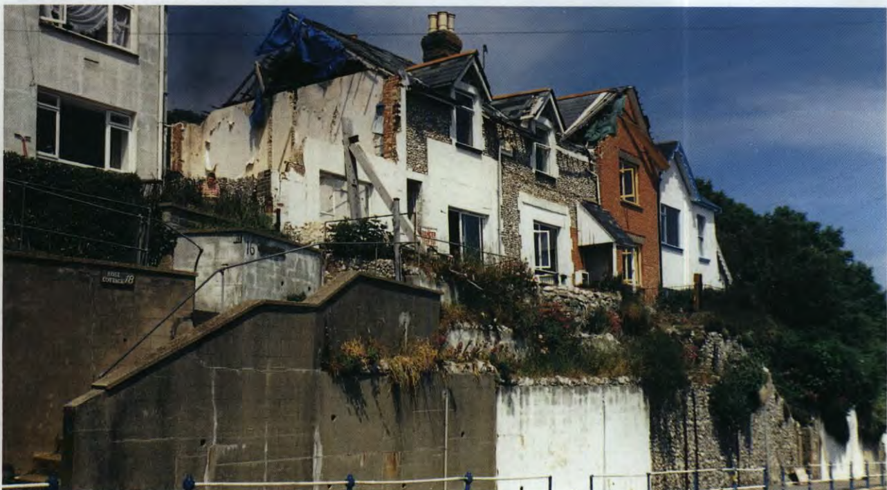
Plate 5: Severely fractured and tilted structure in course of demolition (1988)
