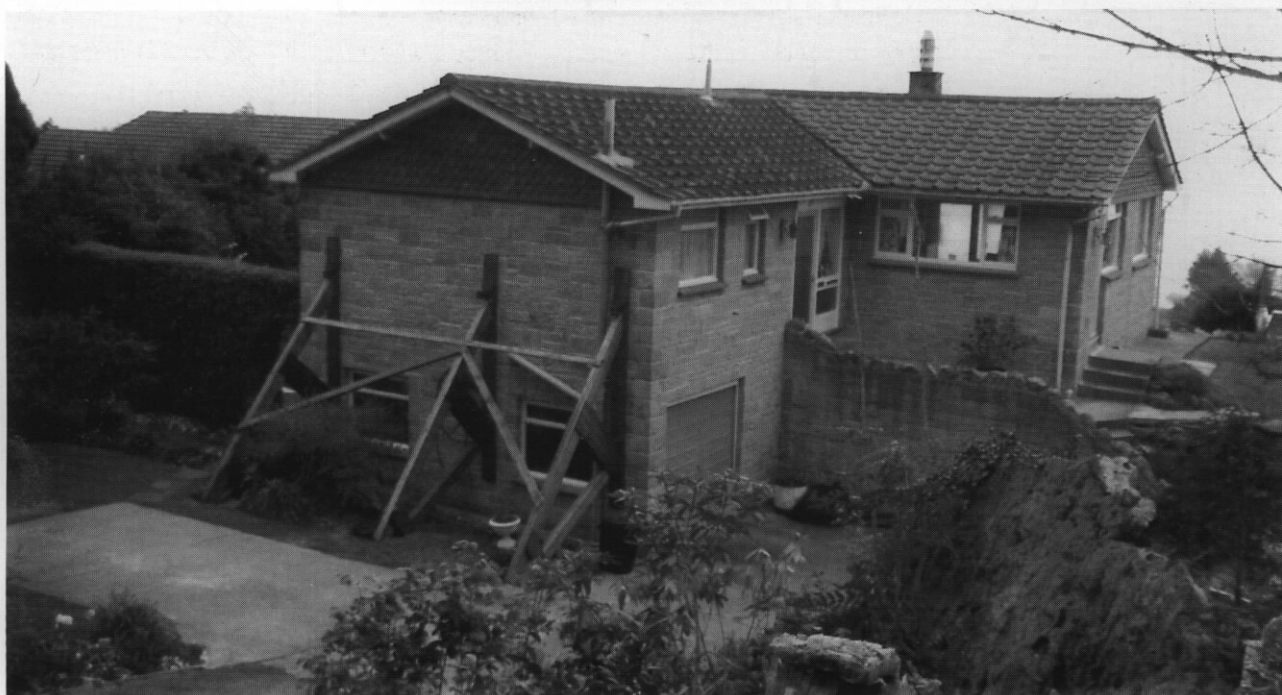
Plate 14: Raking shores used to counter localised rotational tilt
