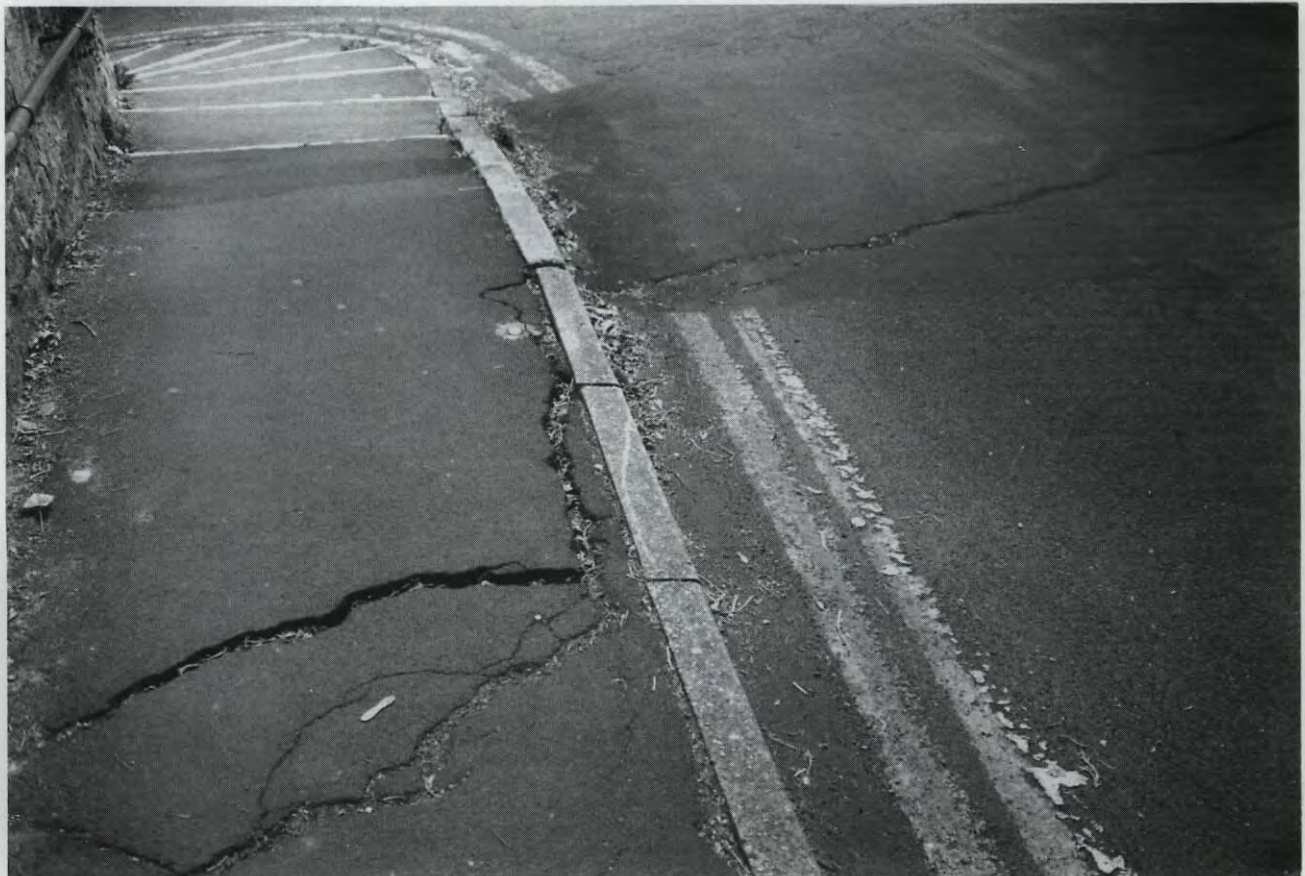
Plate 4: Severe cracking, extension and settlement to the road and footpath
