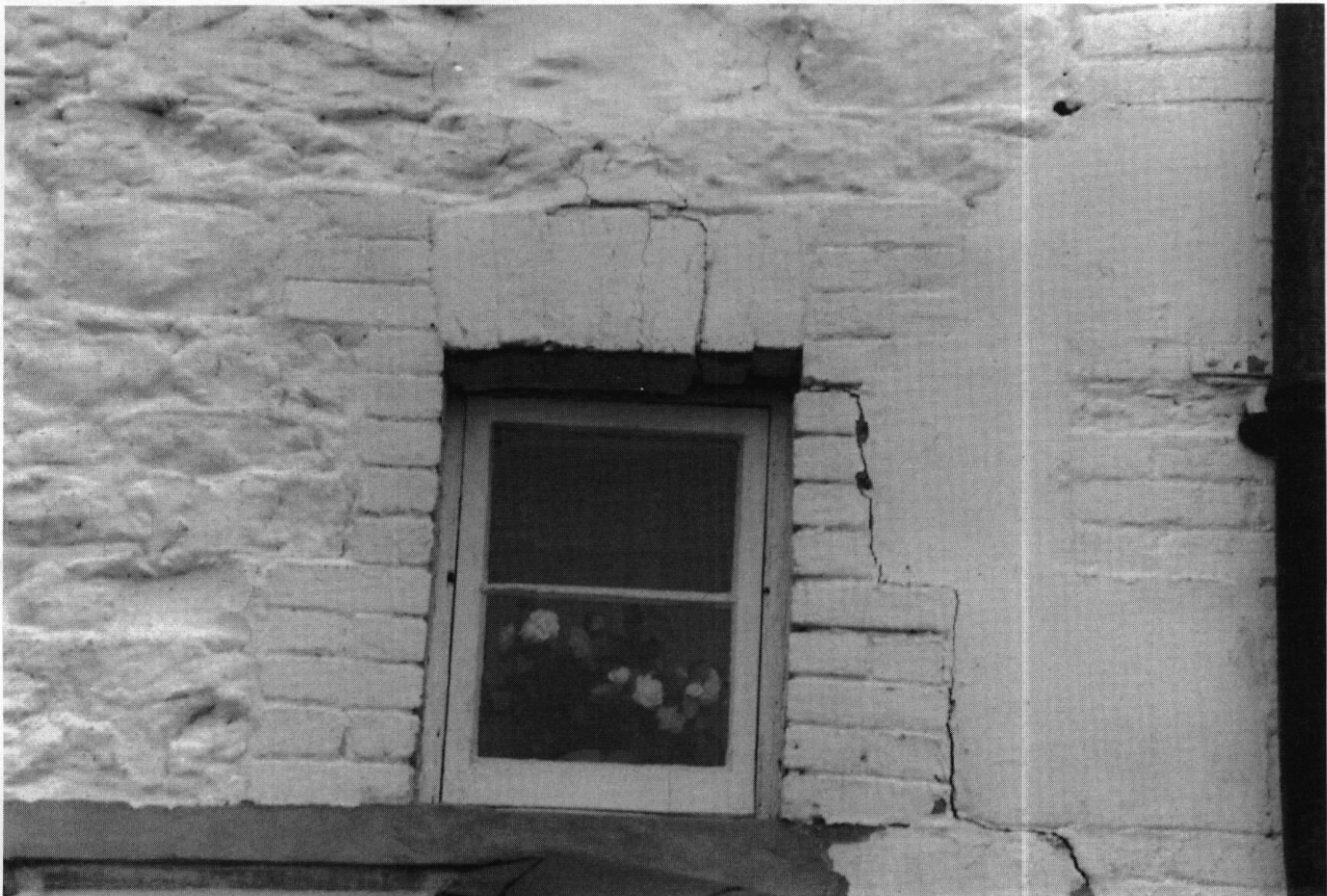
Plate 16: Both long-standing movement and recent fracturing are evident in this photograph
