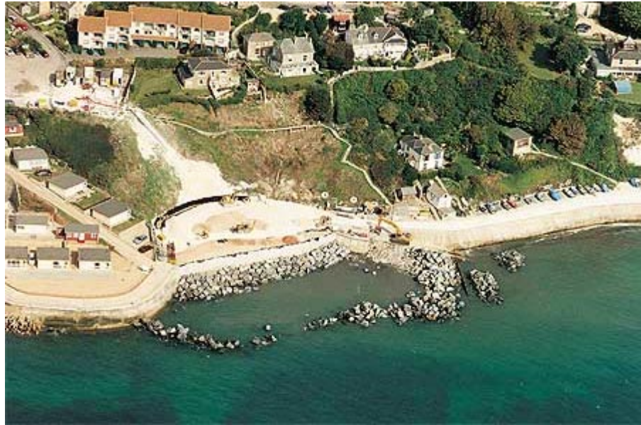
Plate 5a Coast protection and slope stabilization works in progress, 1999 (courtesy:D.Bowie Photography)
