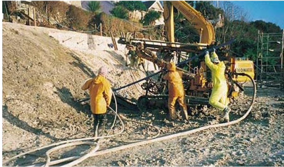
Plate G5c Soil nailing on the upper slope, 1999
