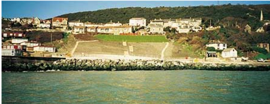
Plate G5e The completed coast protection and slope stabilisation scheme, April 2000
