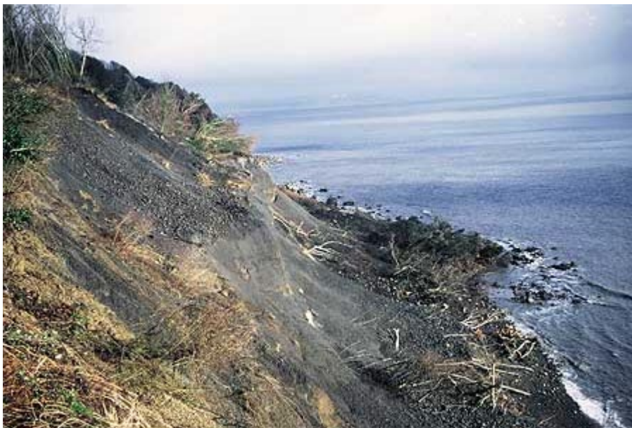
Plate G3b Landslide debris covers the sea, cliff and foreshore
