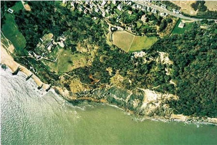
Plate G3a Damage area arising from the 1995 landslide
