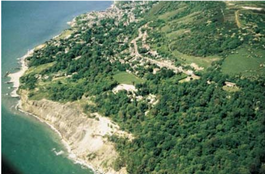
Plate G3 Bonchurch landslide, February 1995, Isle Of Wight , UK
