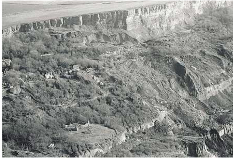
Plate G8a Photo showing the 1994 landslide at Blankgang (County Press)
