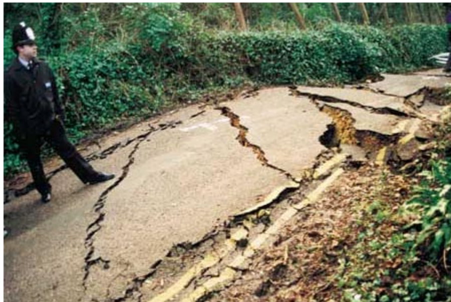
Plate G8e Road damage at Blackgang
