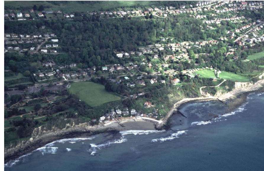
Figure 4: The southern town of Ventnor, part of the largest urban landslide complex in north-west Europe. © IWCCE.
