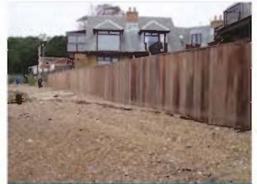
Timber Clad Sheet Pile Wall
