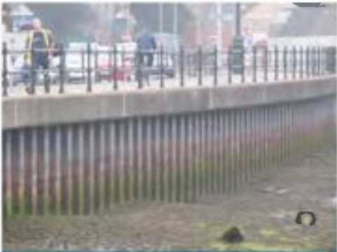
Steel Sheet Piling
