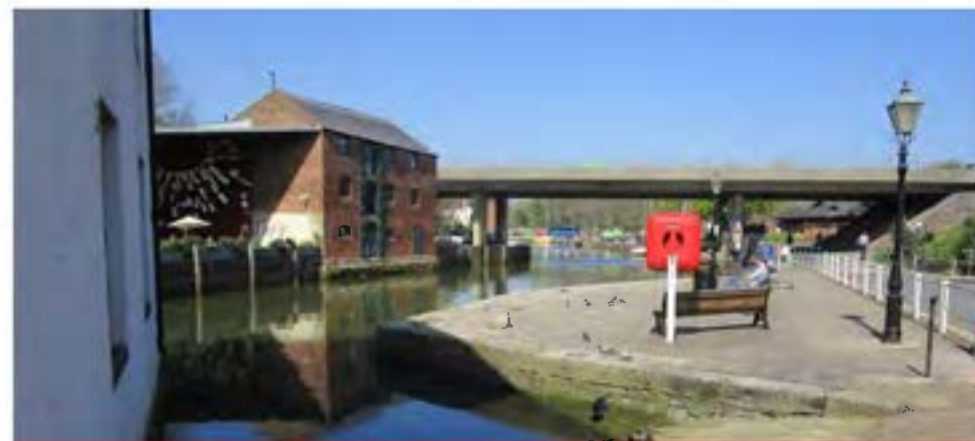
Quay walls of Newport Harbour
