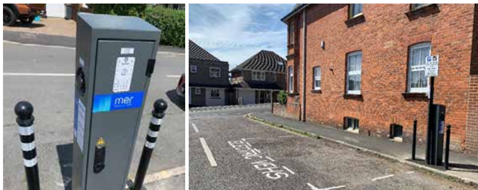
Figure 2: On-street charge point installations as part of pilot project
