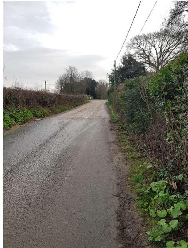
Figure 21: Millfield Avenue, which leads to Holy Cross primary school, has no pavement and could be designated as a low traffic neighbourhood to provide a safer cycling and pedestrian route
