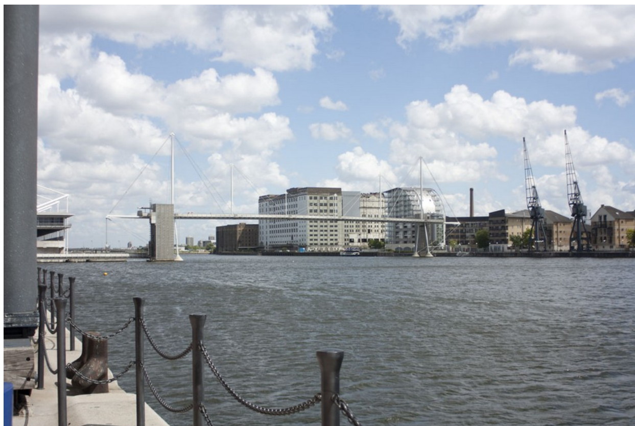
Figure 24: The Royal Victoria Dock Pedestrian Bridge in London was completed in 1998 at a cost of £5 million. This bridge has a span of 127.5 metres, comparable to the width of the River Medina.
