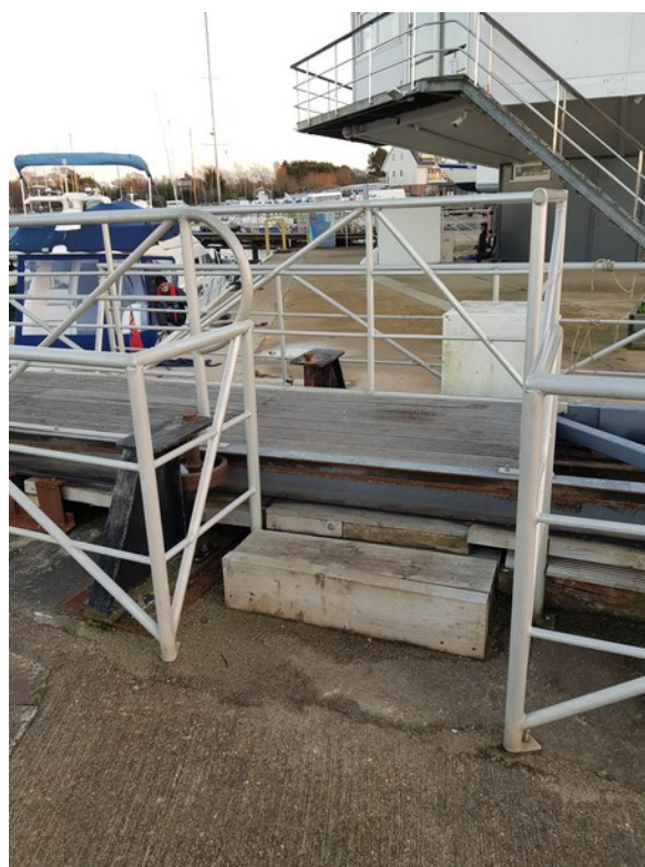
Figure 23: Steps to the lock gate access at Island Harbour
