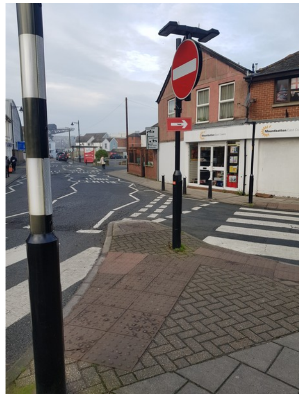
Figure 33: A pinch point at the entrance to Ferry Road in the one-way system leaves little space for a shared use cycle path
