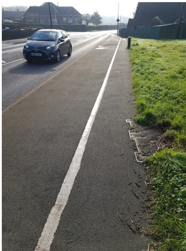
Figure 6: Legacy shared use path with solid white line design on A3021 Whippingham Road is not compliant with current cycle path standards in Local Transport Note 1/20
