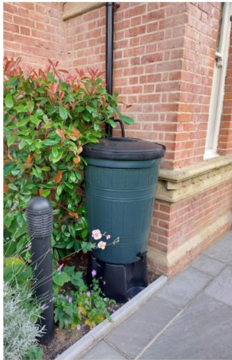
Figure 8-1: Installed slow-drain water butt in Havenstreet (source: Southern Water)
