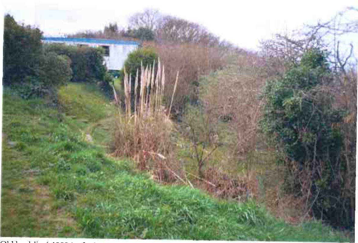
Old landslip (c1980s) of private garden at crest of coastal slope (severe damage)
