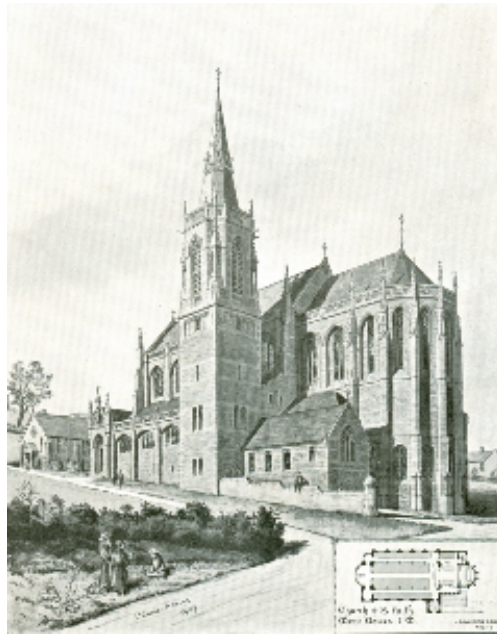
Cowes St Faith – J Standen Adkins Architect (1909)
