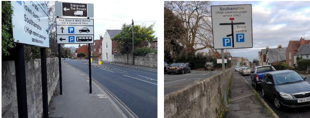
Double pole sign (left) obstructs the footway. Cantilever sign (right) leaves footway clear
