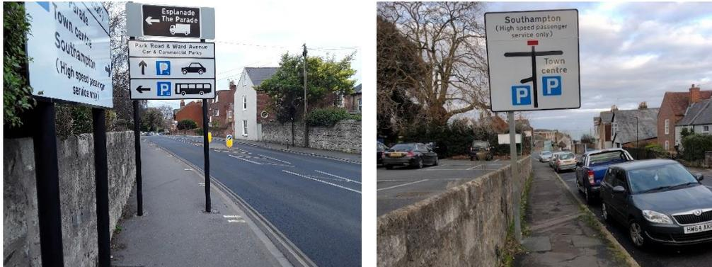
*Double pole sign (left) obstructs the footway. Cantilever sign (right) leaves footway clear*
