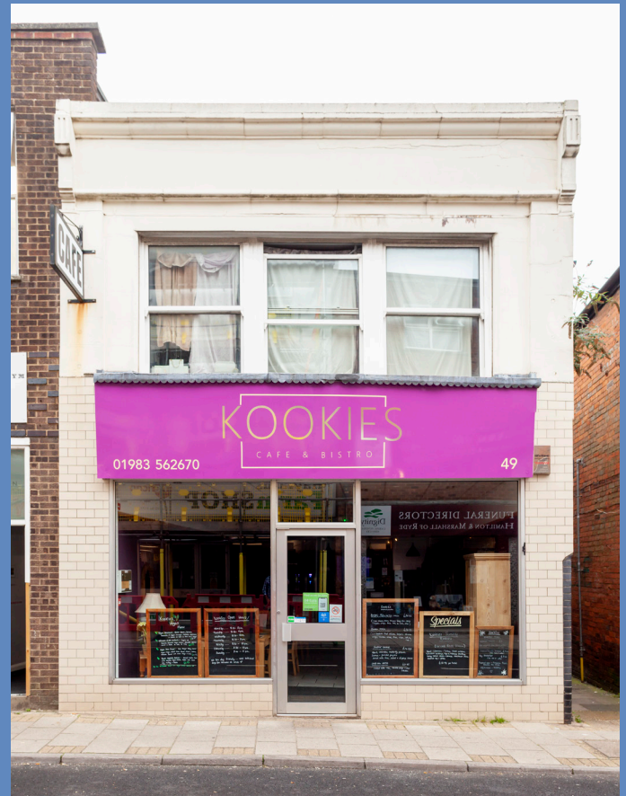
Existing shopfront 49 High Street
