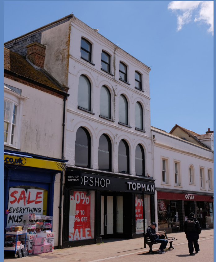
Existing shopfront 20 St James' Square
