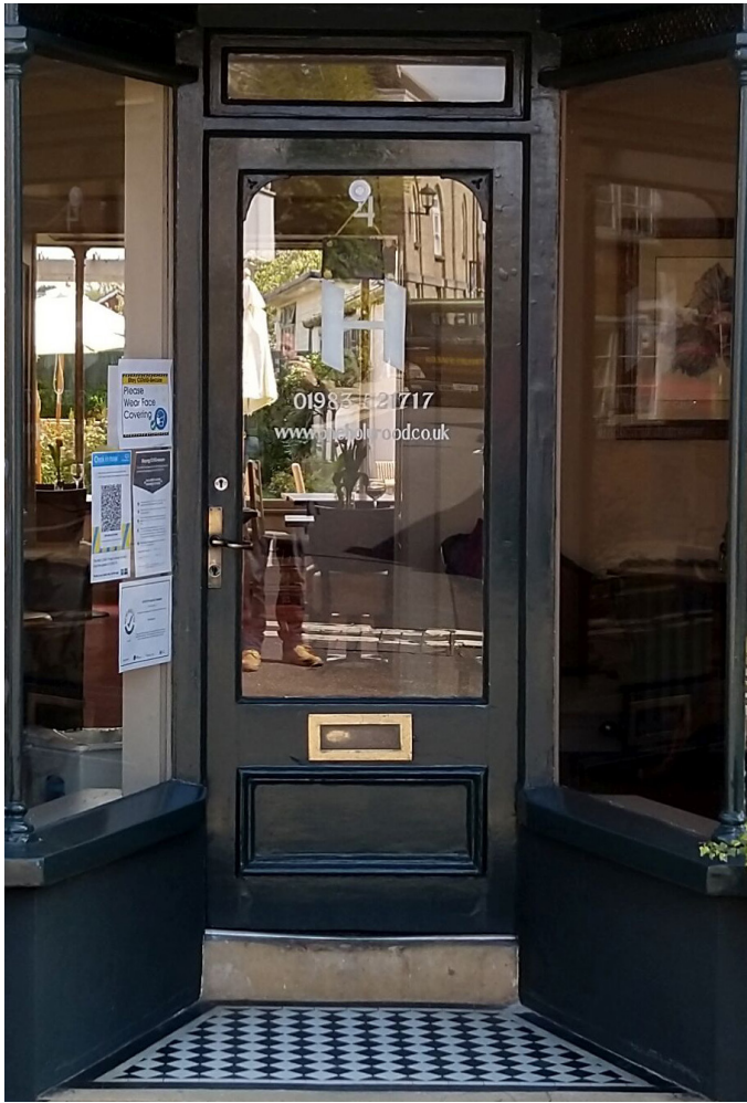
Spandrels used in the top corners of a door's glazing, Newport
