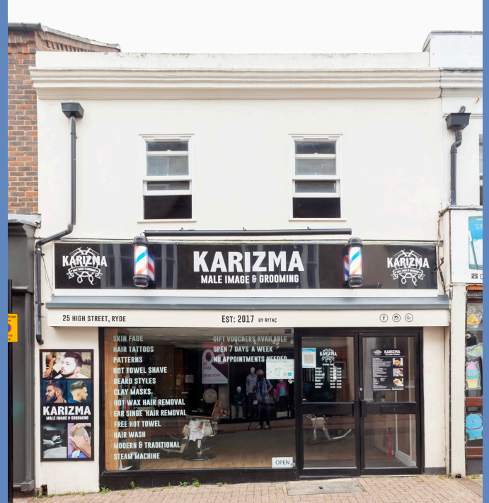
Existing shopfront 25 High Street
