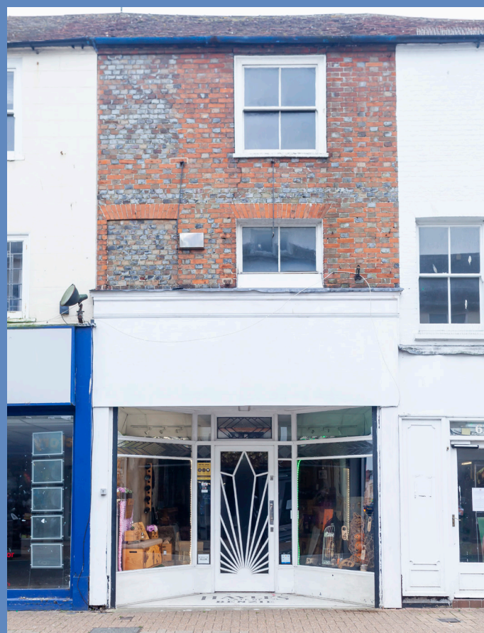
Existing shopfront 60 High Street
