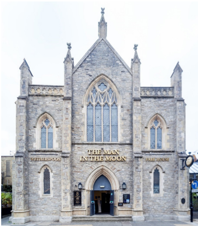
The Man in the Moon is one of the most popular examples of a (now) commercial frontages in Newport according to the survey undertaken in support of this guidance. It reuses the frontage of the former Congregational Church with minimal additions.
