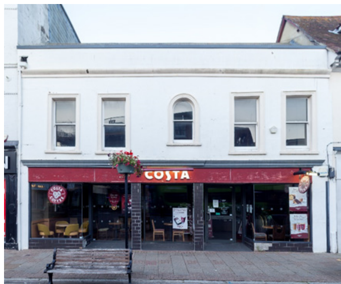
Costa coffee in St James' Square, Newport is an example of a poorly retrofitted shopfront onto a non-standard commercial frontage that used to be a local inn.
