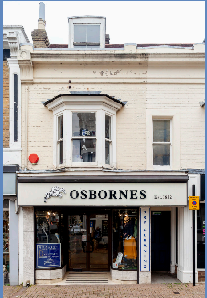
Existing shopfront 29 High Street
