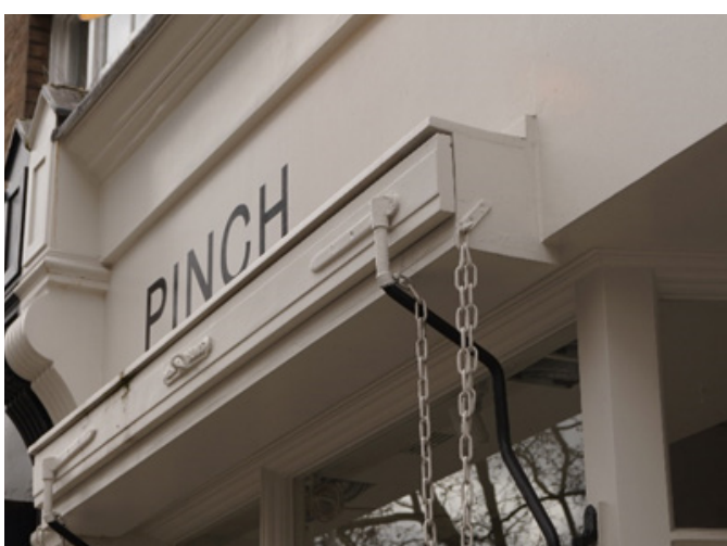
A good example of a blind that is not integrated into shopfront, London
