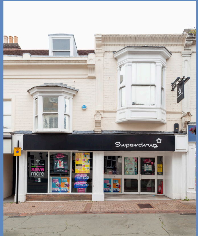
Existing shopfront 30-31 High Street
