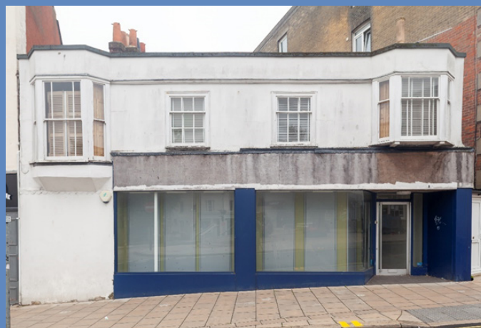
Existing shopfront 9 St Thomas' Square
