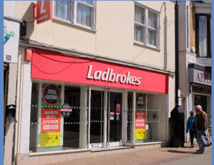
Existing shopfront 27 High Street
