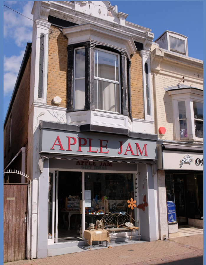
Existing shopfront 28 High Street
