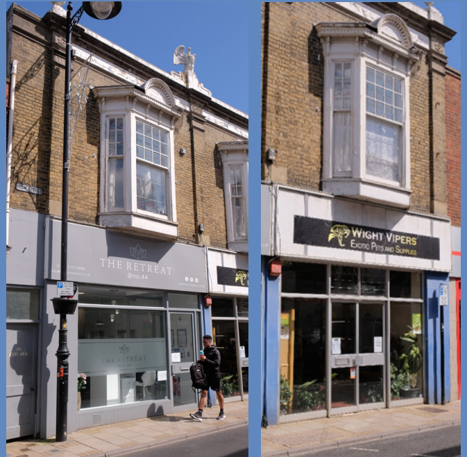
Existing shopfronts 44-45 High Street
