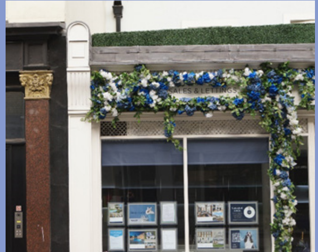
An example of excessive greenery that obscures the view of the fascia
