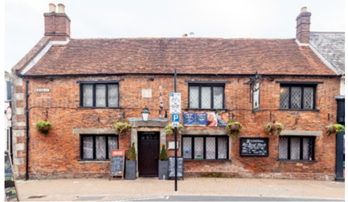
A non-standard commercial frontage in a 17th century building, The Castle Inn, Newport
