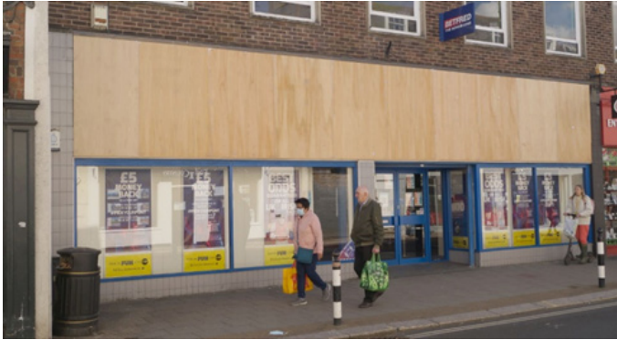
A poor example of an excessive fascia in Newport where the fascia makes up about 50 per cent of the entire shopfront. This makes the shop look like a billboard rather than a commercial premises.
