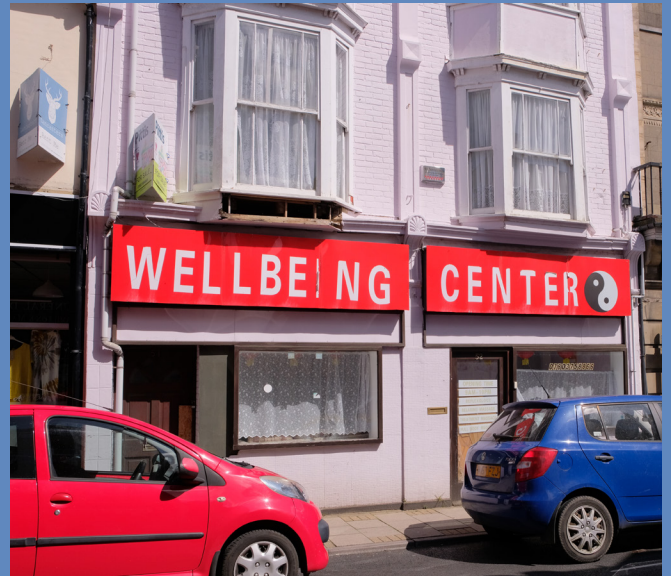
Existing shopfront 51-52 High Street
