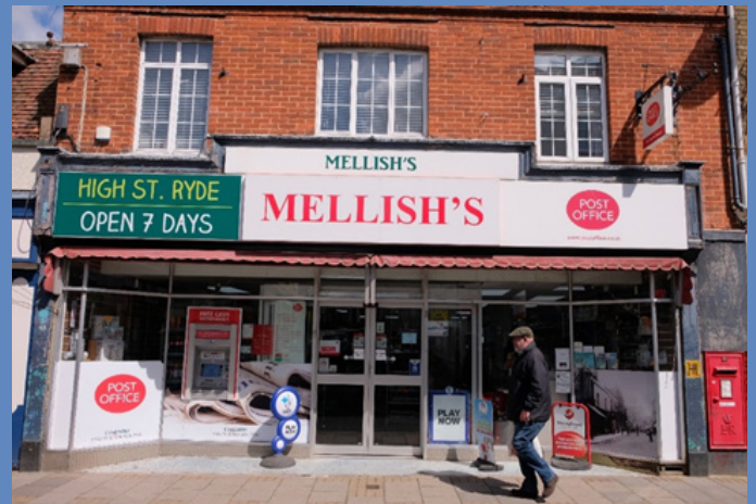
Existing shopfront 43 High Street
