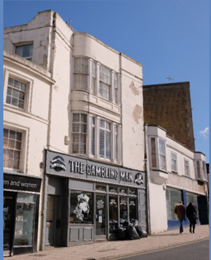
Existing shopfront 5 St Thomas' Square
