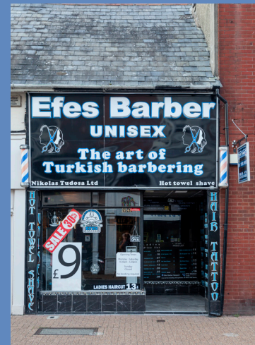
Existing shopfronts 92-94 High Street
