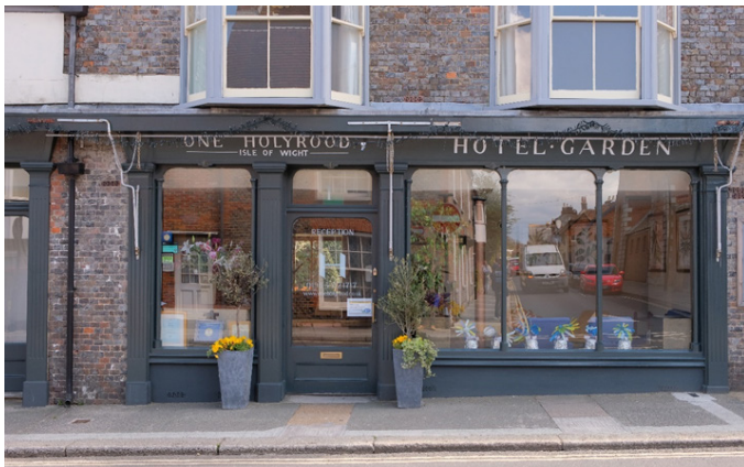
A Georgian style shopfront in Newport
