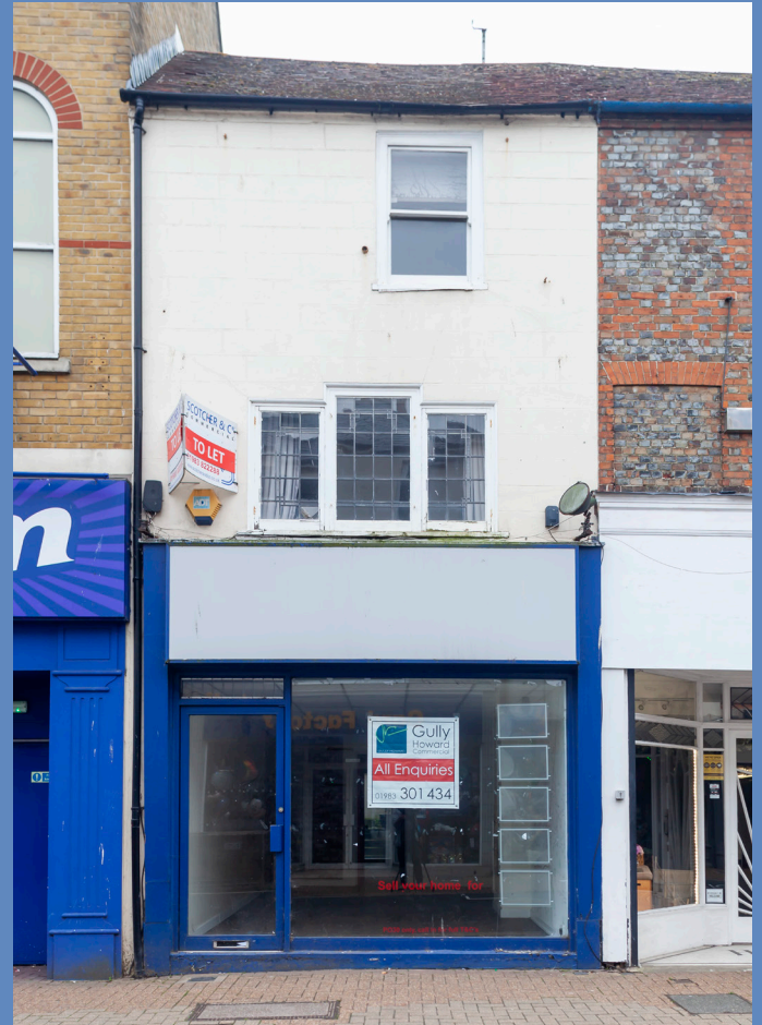
Existing shopfront 59 High Street
