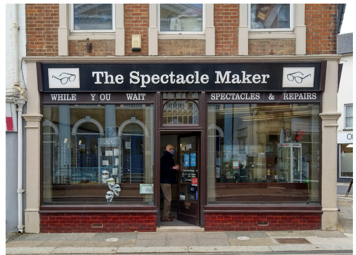
An example of a shopfront with clear and effective signage and advertising that keeps the shop windows free from clutter
