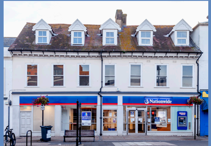
Existing shopfront 22 St James' Square
