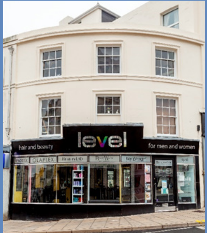
Existing shopfront 4 St Thomas' Square
