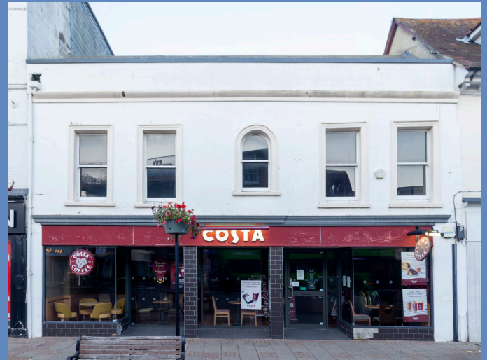
Existing shopfront 21 St James' Square
