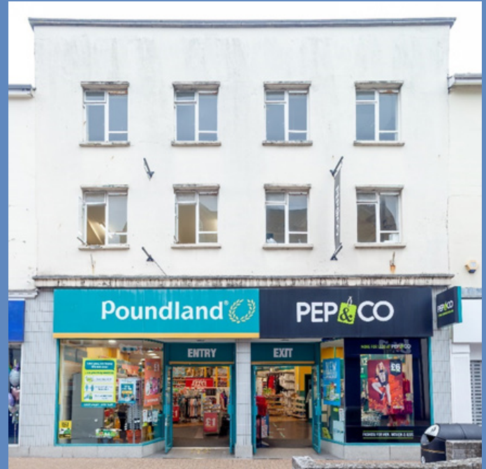
Existing shopfront 104 High Street
