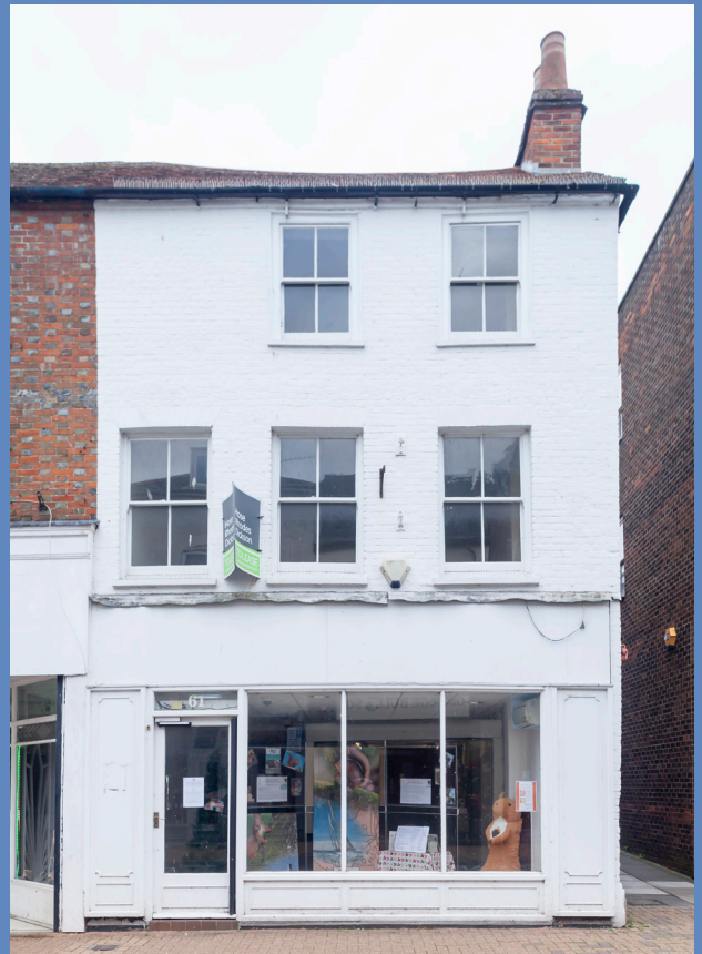
Existing shopfront 61 High Street
