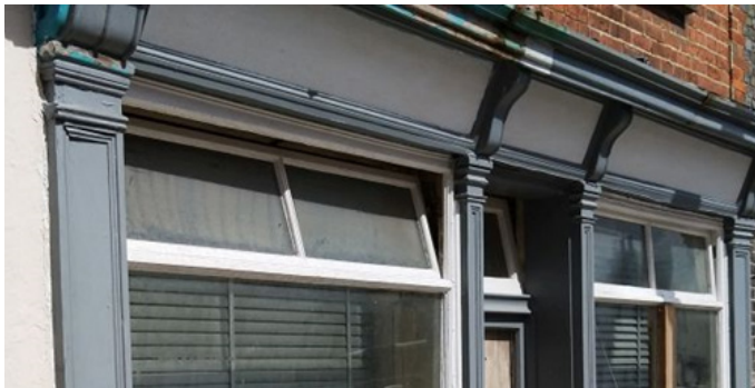
A 'hopper opening' transom light, Newport
