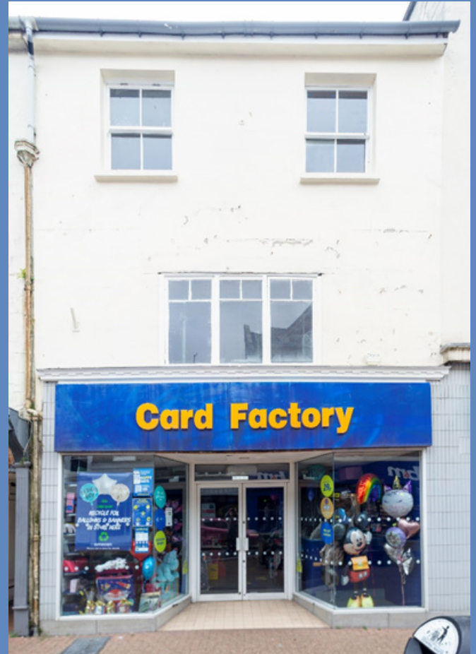
Existing shopfront 103 High Street
