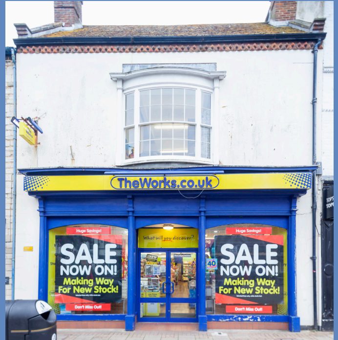
Existing shopfront 19 St James' Square
