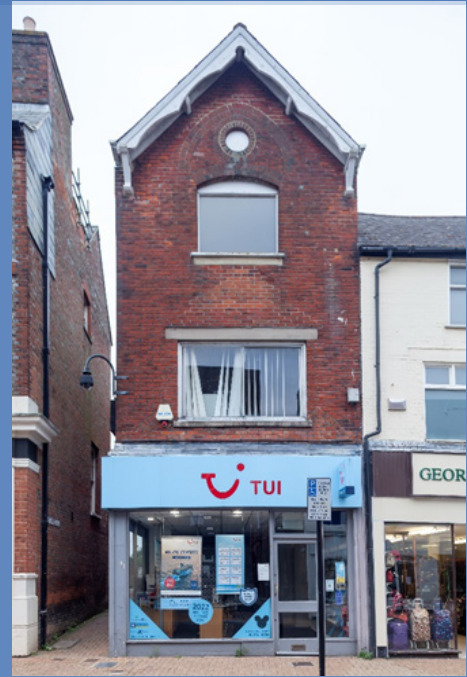
Existing shopfront 100 High Street
