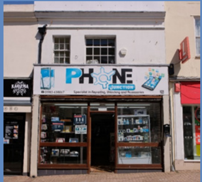
Existing shopfront 26 High Street
