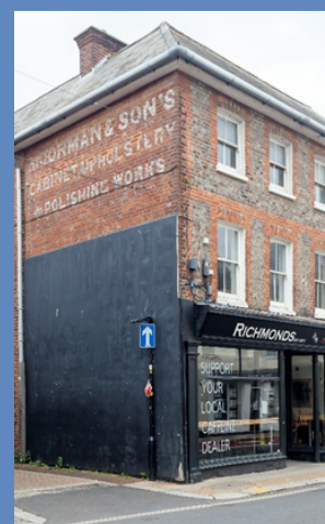
Existing painted sign on the side of a nearby building in St James' Square, Newport
