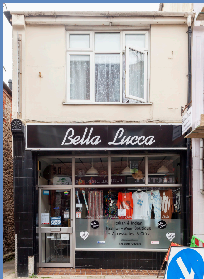
Existing shopfront 50 High Street
