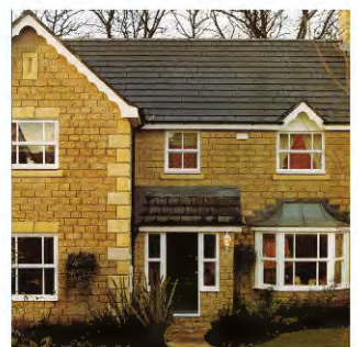
Avoid uniform units of reconstructed stone.
