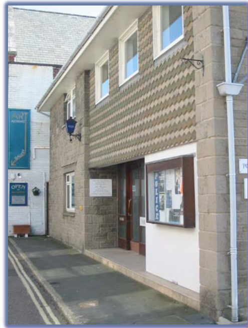
Yarmouth Police Station © BCE
