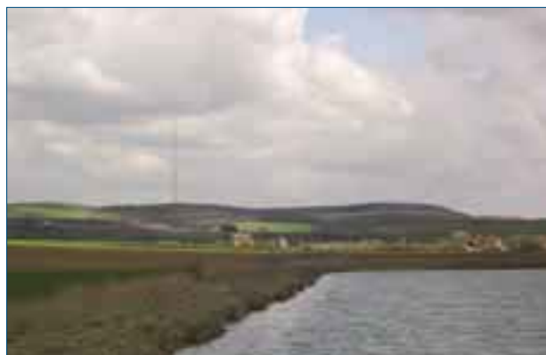
Storage reservoir at Atherfield
