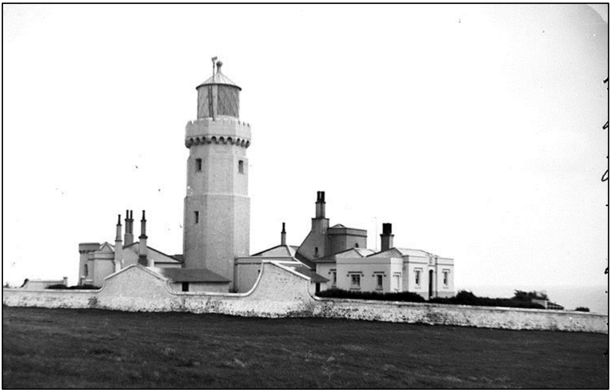
St. Catherine's Lighthouse. A view of St. Catherine's Lighthouse situated at Niton Undercliff. The white octagonal tower has 94 steps up to the lantern. Circa. 1890-1914
